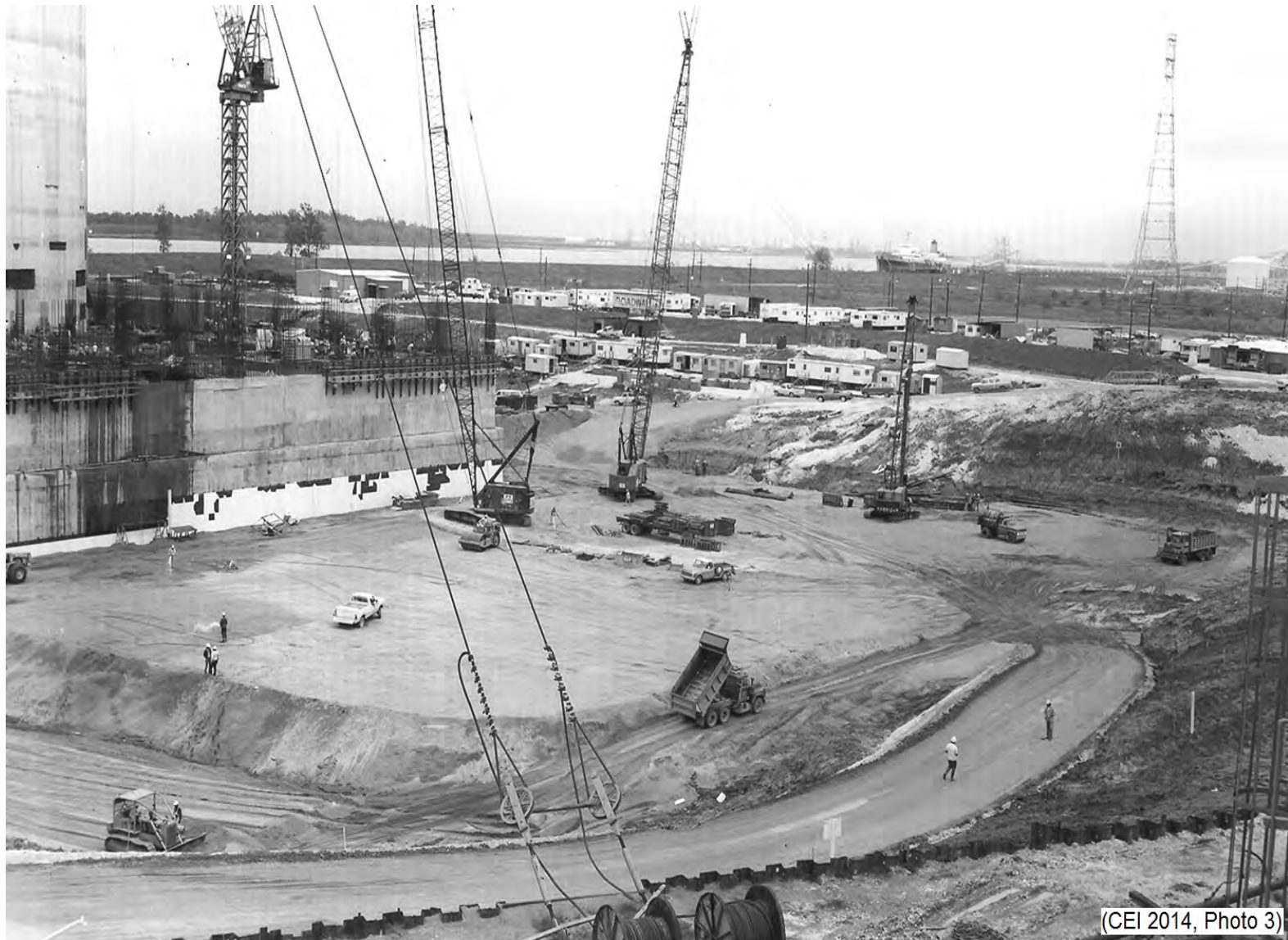
Figure 3.7-11 WF3 Plant Construction, 1978
