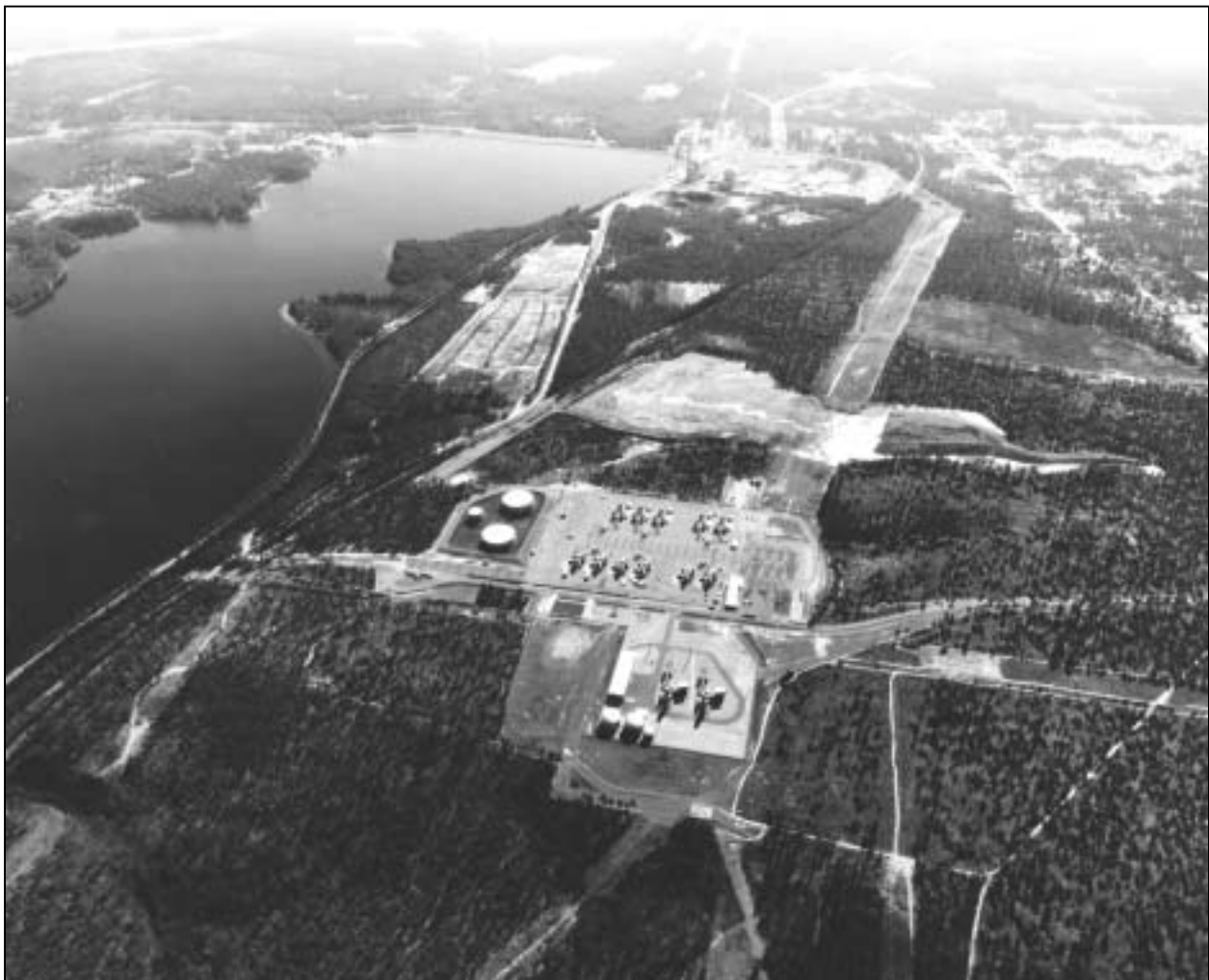
View looking South. Darlington County plant in foreground, Lake Robinson to left, and Robinson Steam Electric Plant in background.
