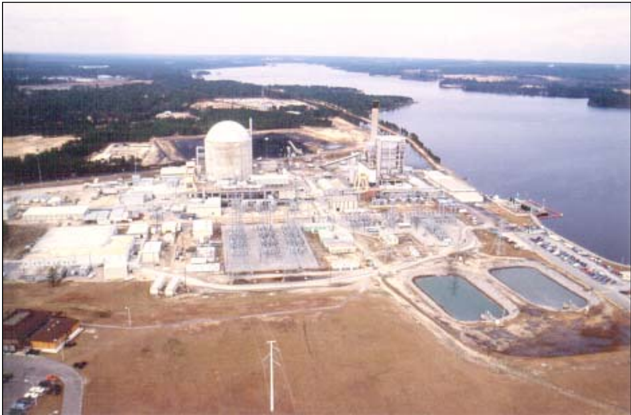
Robinson Nuclear Plant and Lake Robinson
