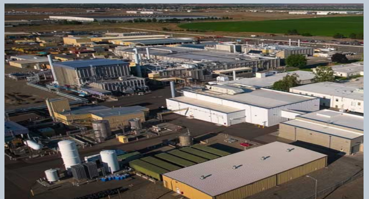
Framatome, Inc. Fuel fabrication facility in Richland, Washington. Photo Courtesy of Framatome, Inc.
