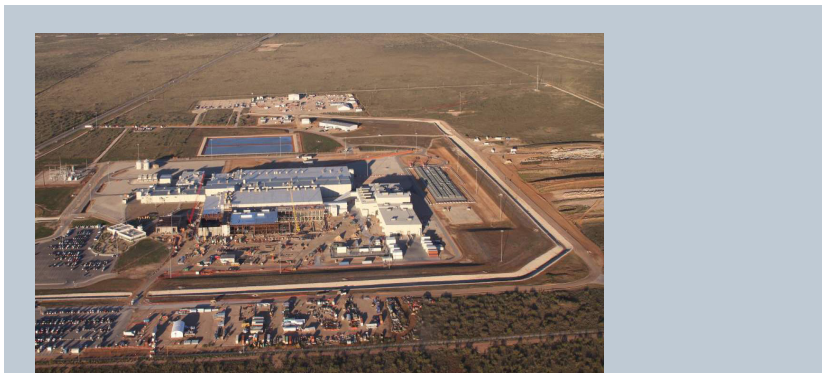
URENCO USA facility in Eunice, New Mexico.
