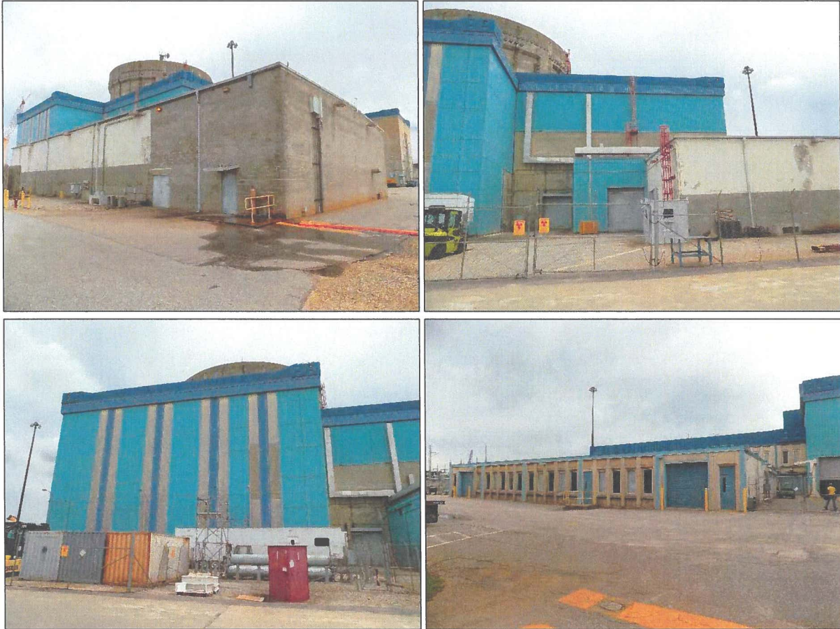
Figure 12. Representative view of 0116–Nuclear Reactor Complex (Summer 1). Top left: radioactive materials building, facing east. Top right: hot machine shop, facing south. Bottom left: fuel handling building, facing south. Bottom right: services building, facing southwest.
