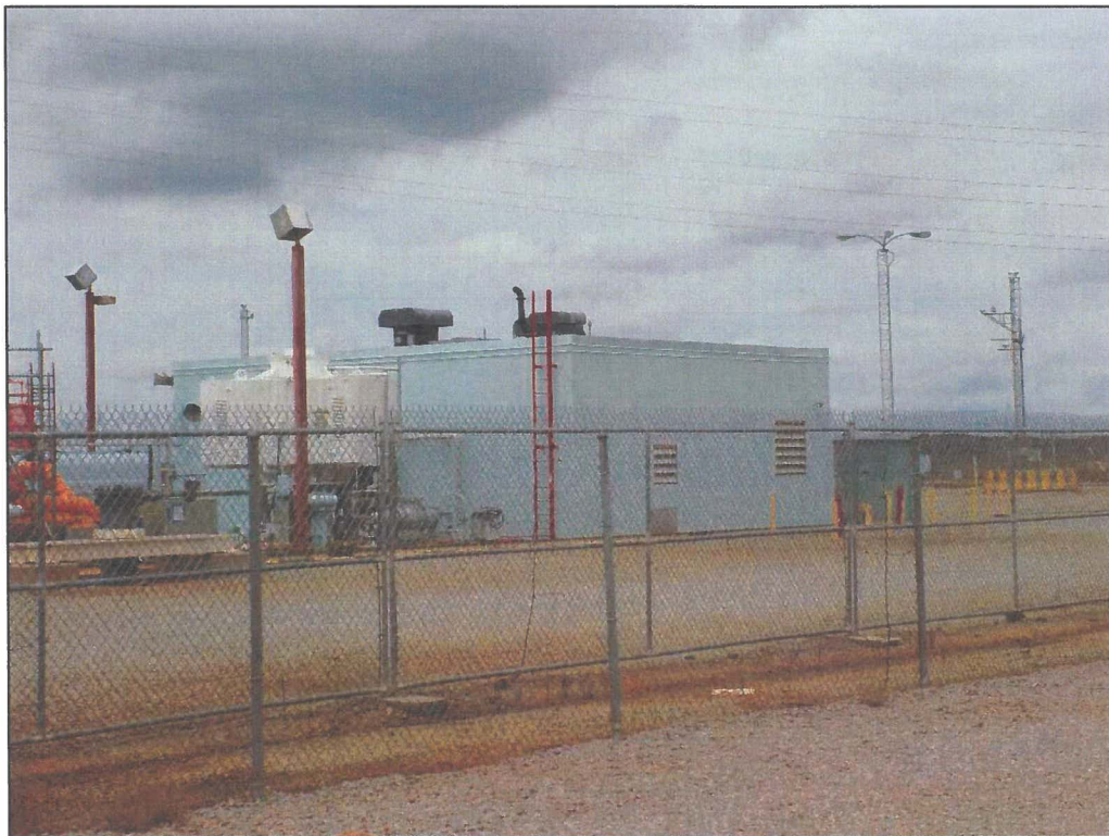
Figure 18. Building 0121, facing northeast.
