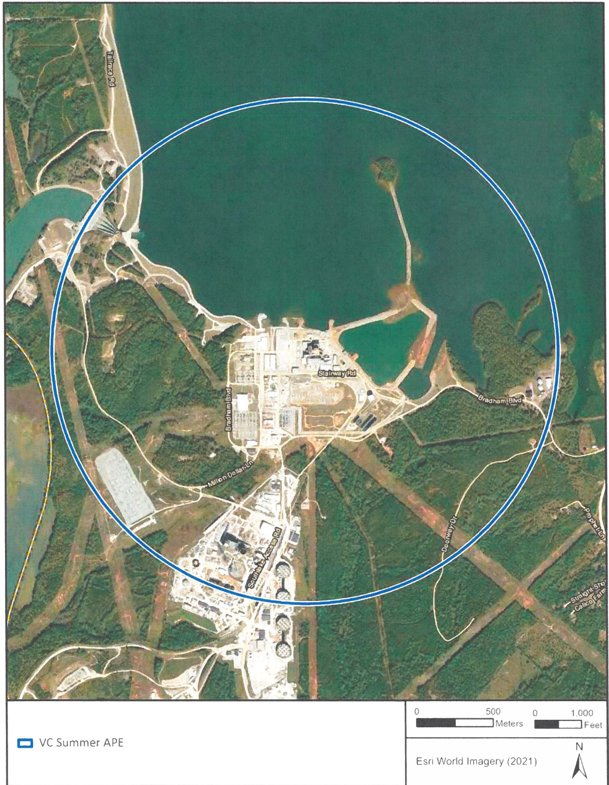
Figure 2. The VCSNS APE in Fairfield County, South Carolina.
