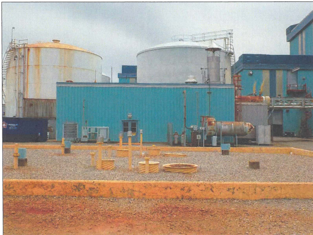
Figure 21. Building 0124, facing south.
