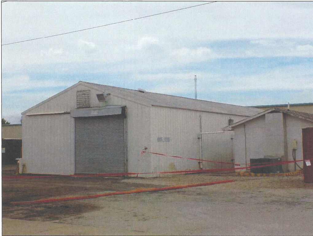
Figure 34. Resource 0137, facing southwest.
