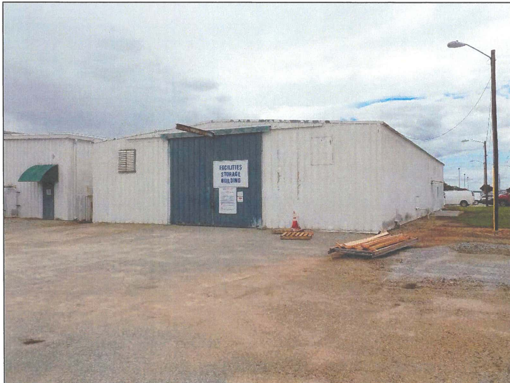
Figure 40. Resource0143, facing southwest
