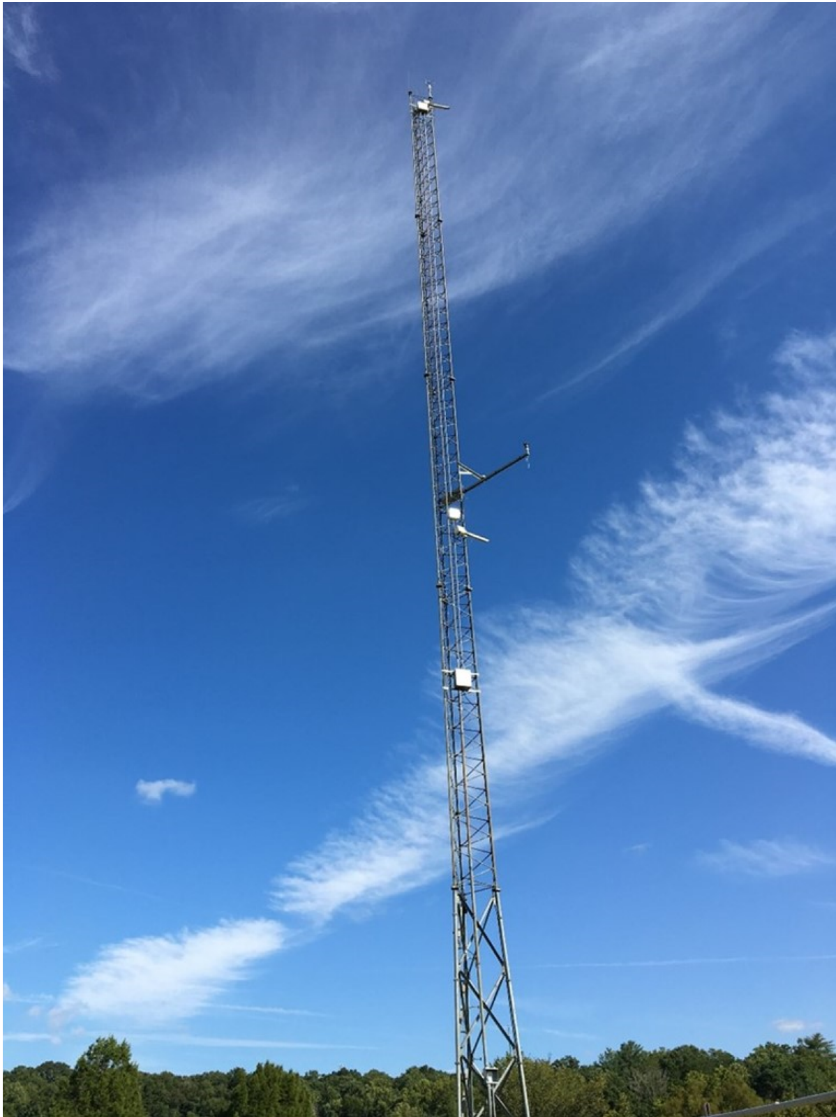
Figure 2.3-25: Photo of Tower L with Wind Measurements at 15 and 30 Meters
