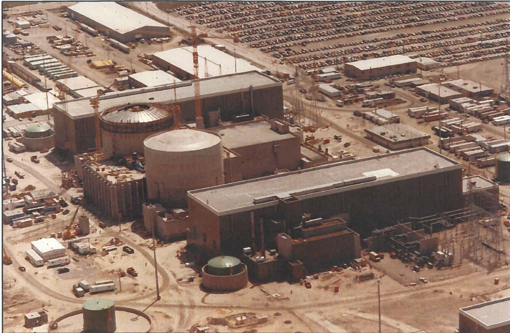
Figure 3.8-9 Construction Photograph of the PNPP Site, May 1983
