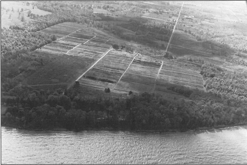
Figure 3.8-4 Preconstruction Photograph of the PNPP Site, October 21, 1974
