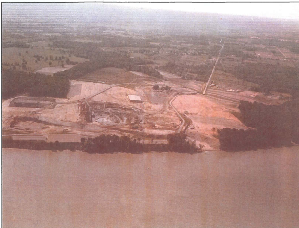
Figure 3.8-5 Construction Photograph of the PNPP Site, September 1975
