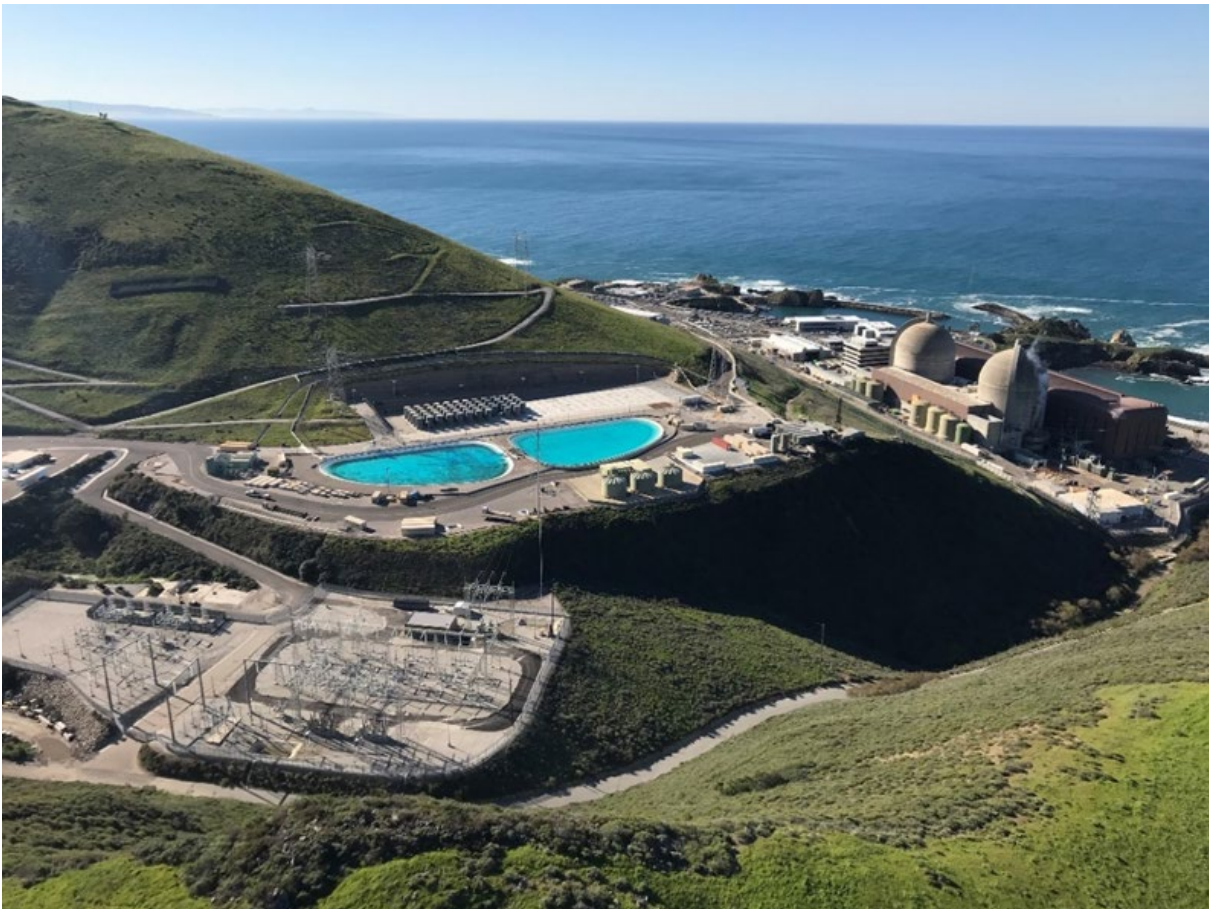
DCPP ISFSI Pad within hillside, on south side of the make-up water reservoirs
