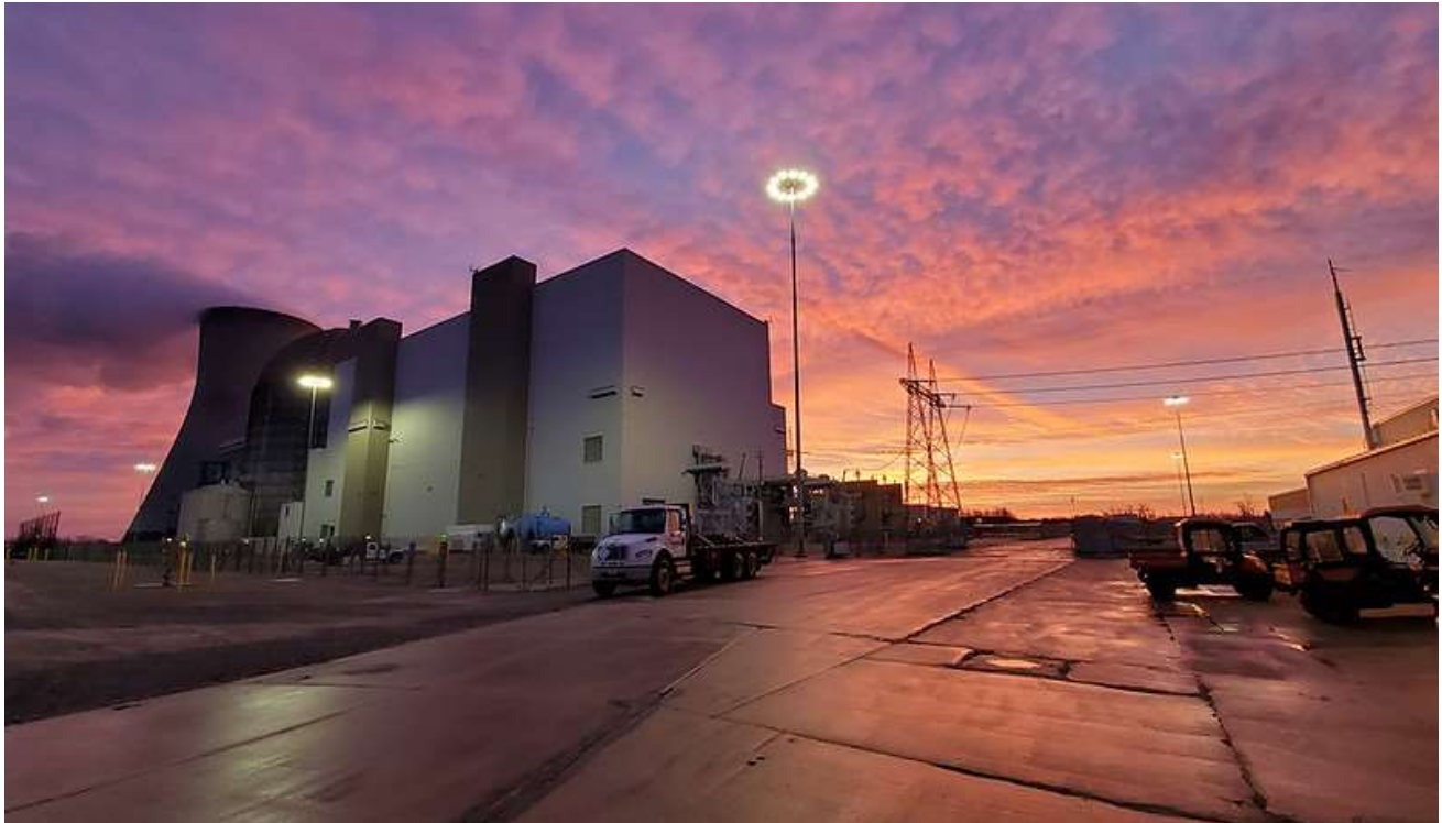
Callaway Nuclear Generating Station
