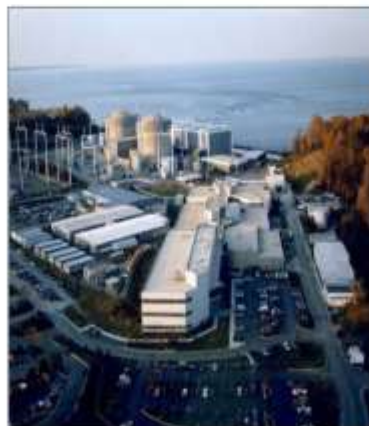
Calvert Cliffs Nuclear Power Plant, Lusby, MD
