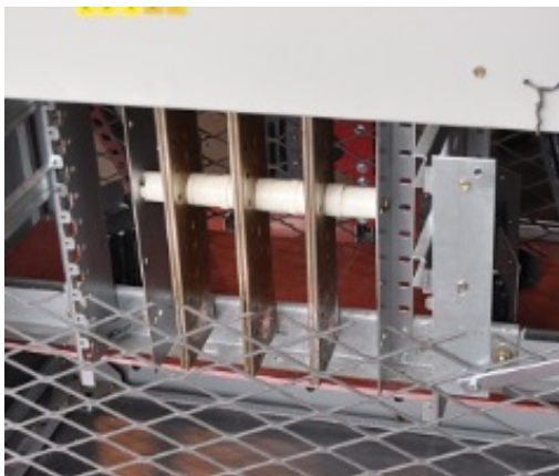
Figure G-1 DP Bus Bar Configuration
