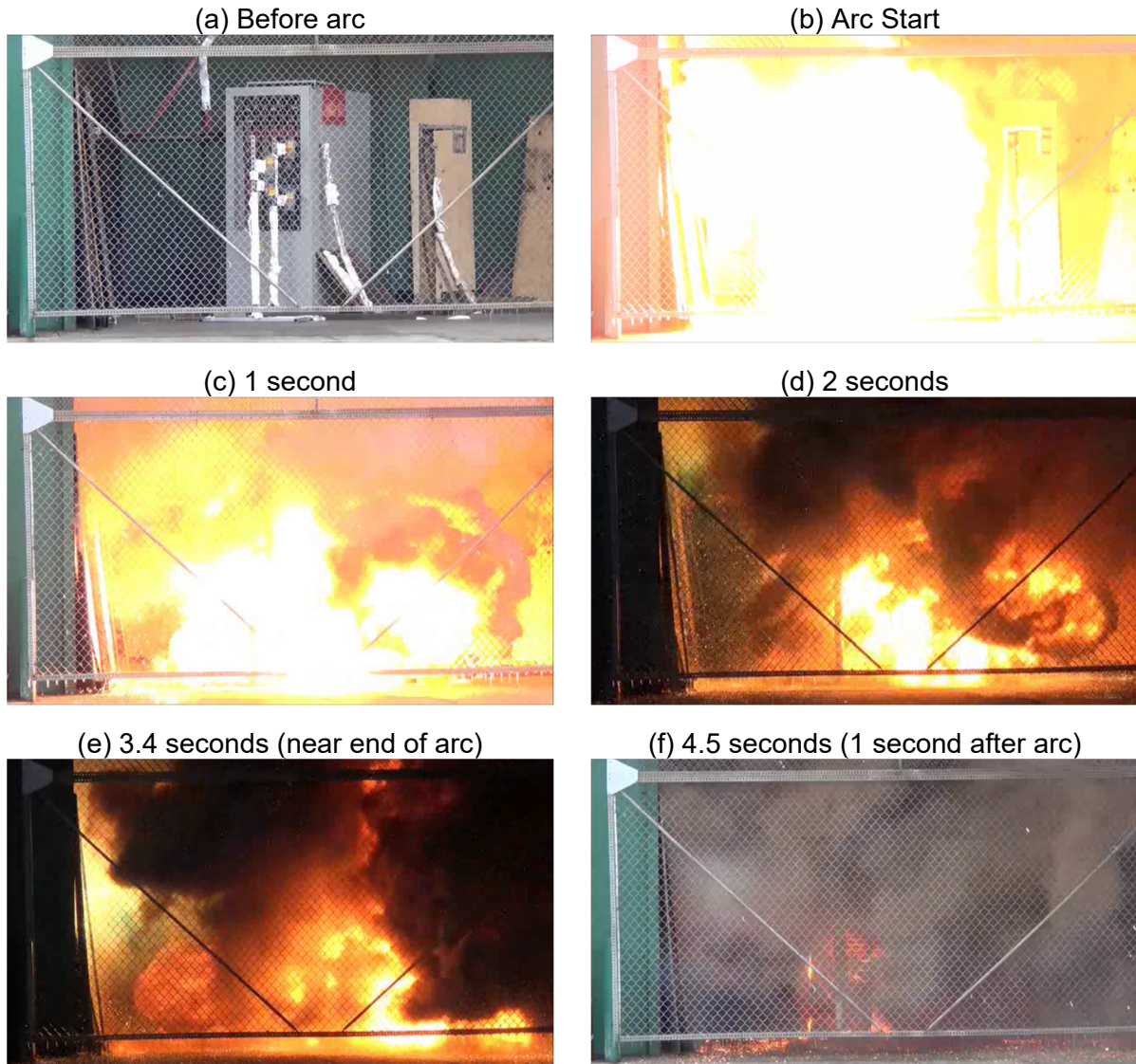
Figure 3.10-1 SWGR Test 8 Arc
