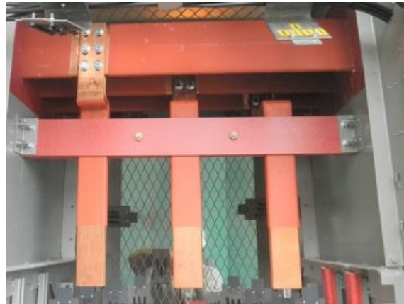
Figure G-2 SWGR Bus Bar Configuration
