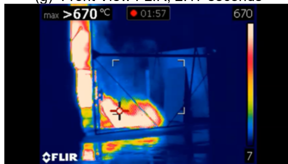
Figure 3.8-2 SWGR Test 7 Flames during Arc
