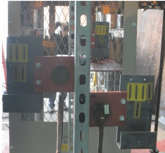
Figure 3.6-1 SWGR Tests Exterior Target Details
