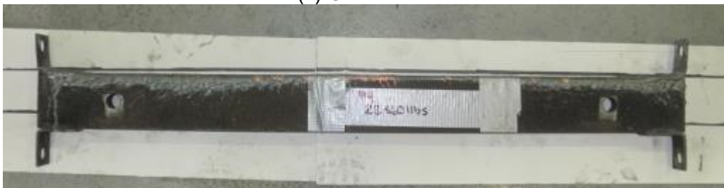
Figure 3.12-7 SWGR Test 10 Bus Bar and Ground Bar Damage
