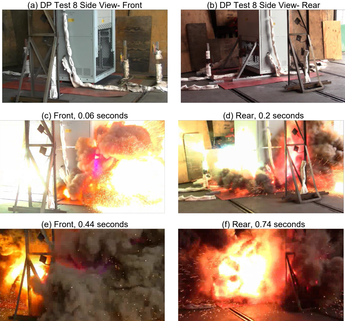
Figure 2.9-2 DP Test 8 Flames during the Arc
