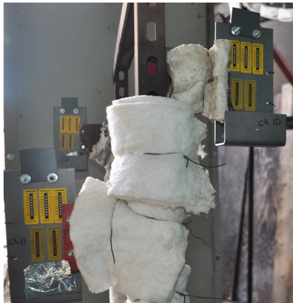
(c) E7-E10 from rear (no damage)
