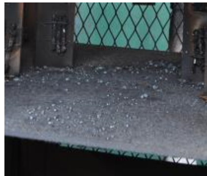
Figure 4.5-1 Metal Sputtering and Coating
