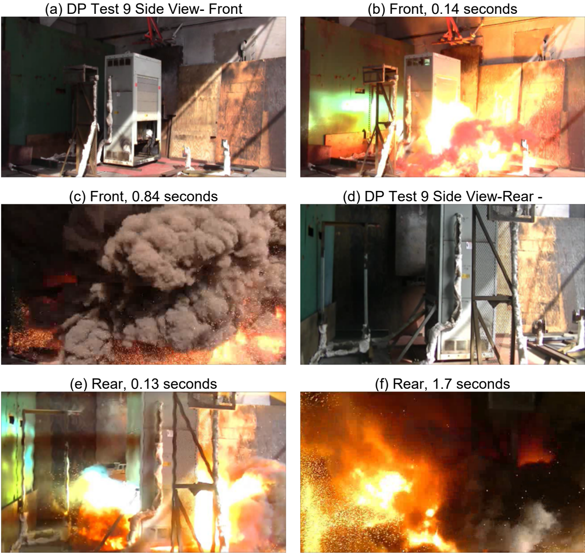
Figure 2.11-2 DP Test 9 Flames During Arc
