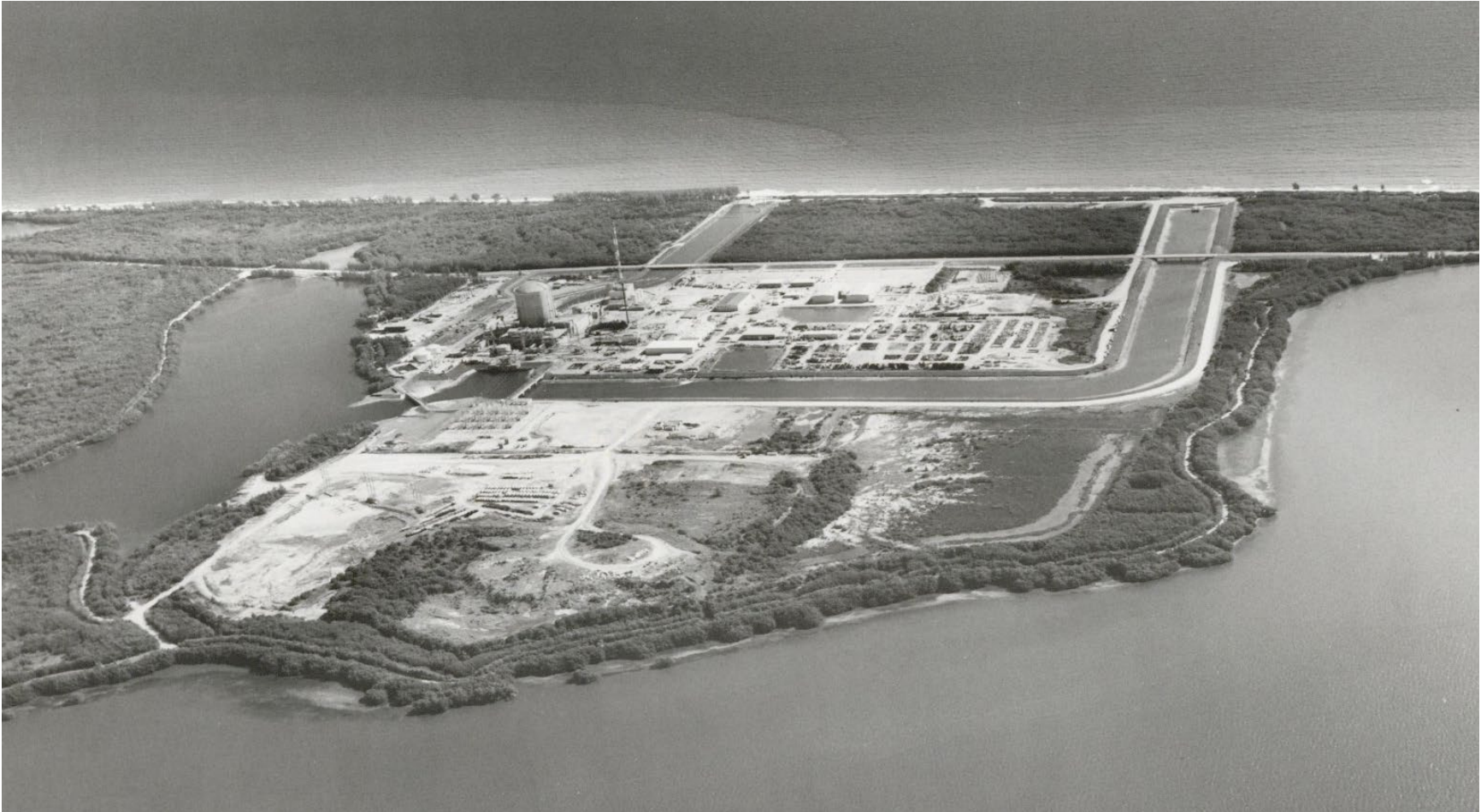
Figure 3.8-8 A Late-State Construction Photograph of PSL Showing Structures, Facilities, Buildings, and the Site Surrounded by Mangroves, the Indian River, and the Atlantic Ocean
