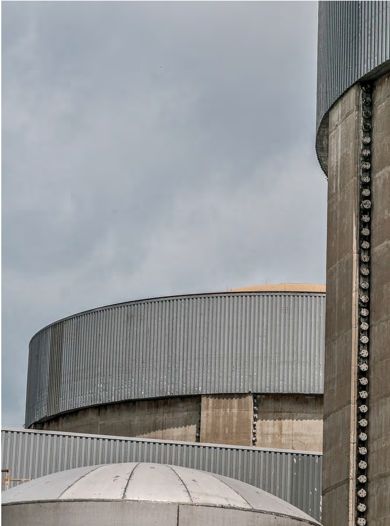
Reactor containment building.
