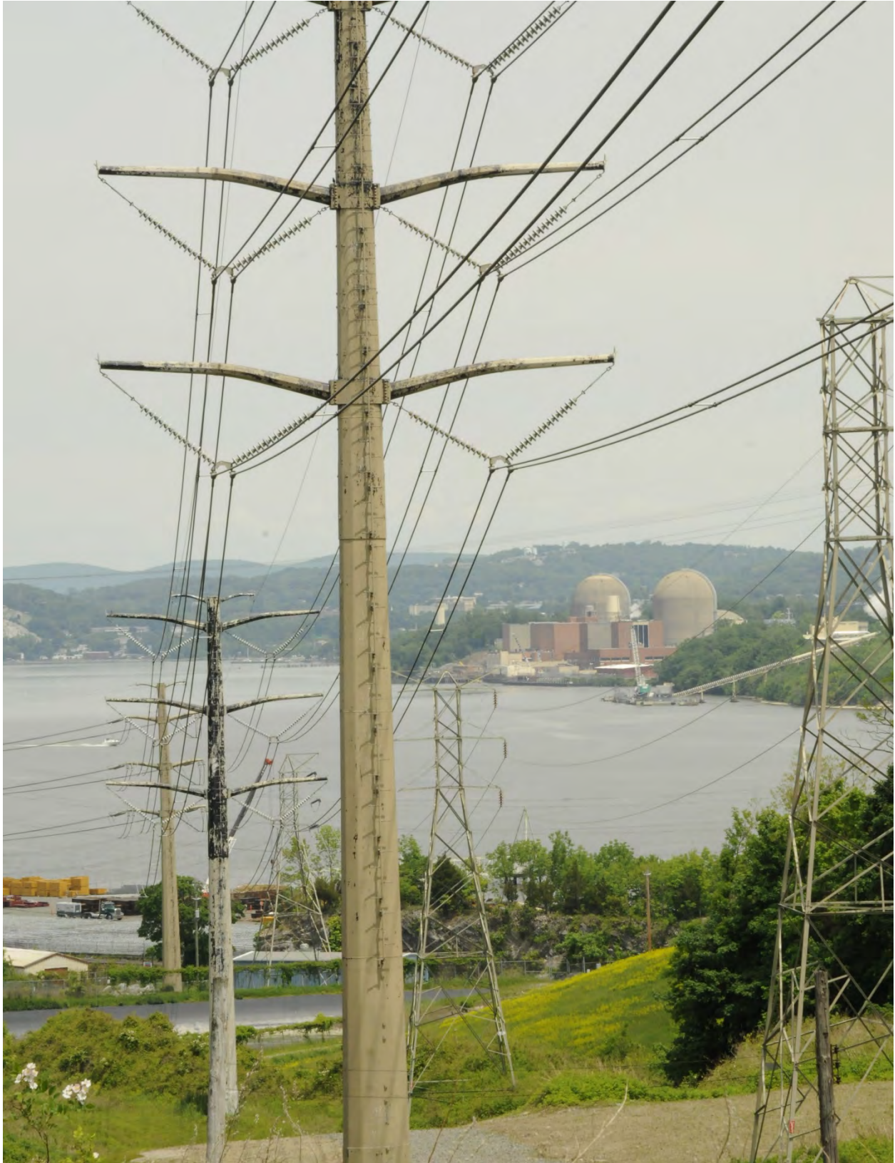
Power lines from Indian Point Nuclear Power Station in Buchanan, New York.
