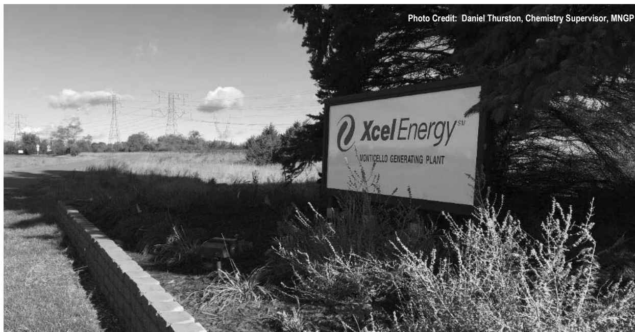
Welcome to Monticello Nuclear Generating Plant
