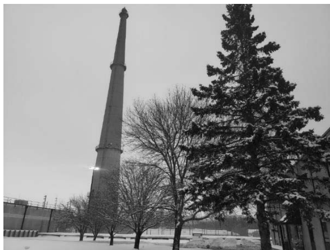
Photo Credit: Daniel Thurston, Chemistry Supervisor, MNGP
