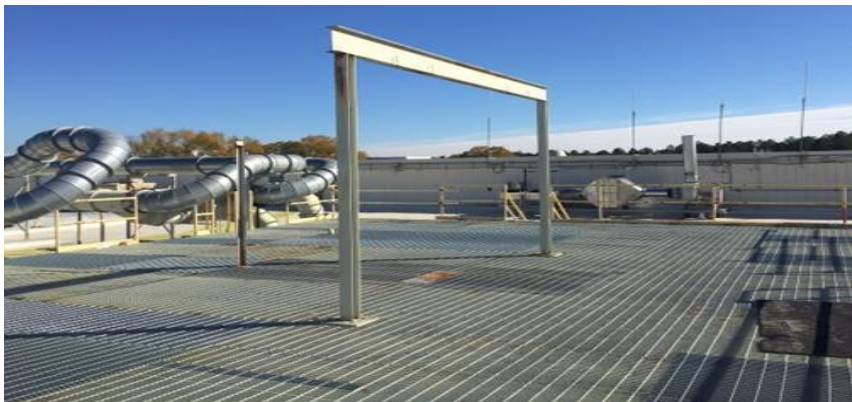
Roof Equipment - After
