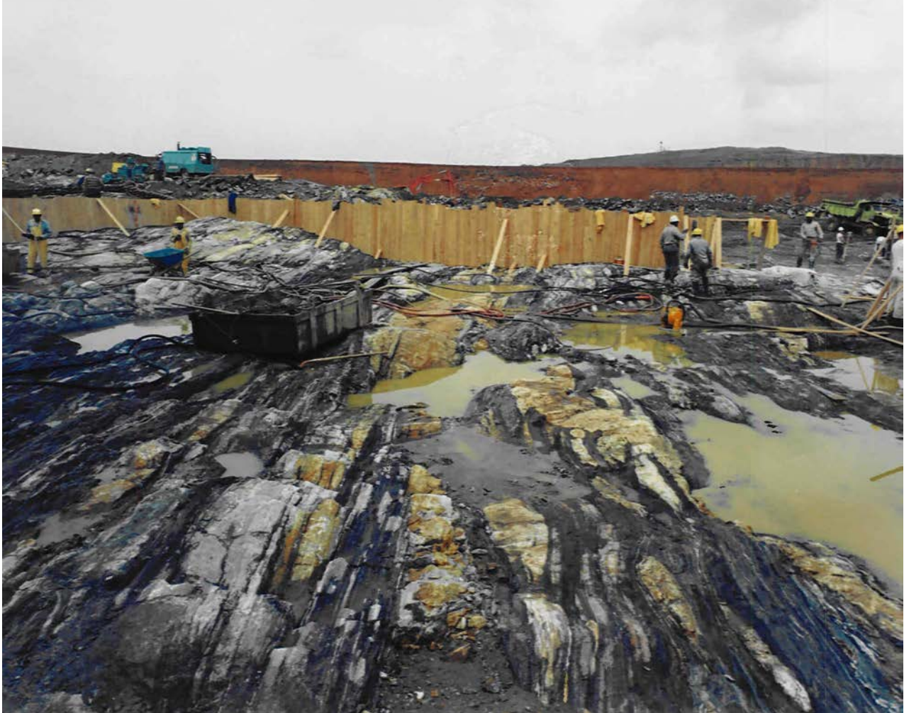
Figure E3.8-14 Construction Photograph of NAPS
