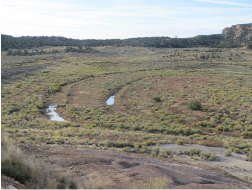
Figure 4: Ponding on the existing disposal cell cover at the Church Rock Site after a rainfall event in 2015.
