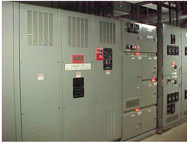
Figure 4: Dry-Type Load Center
