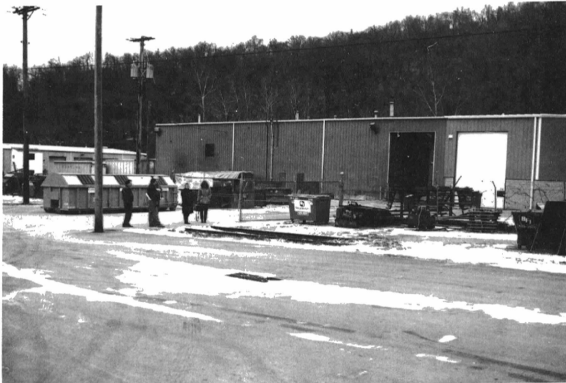
Figure 2.22 Location of Radioactive Source Recycle Container at BFI – Carnegie
