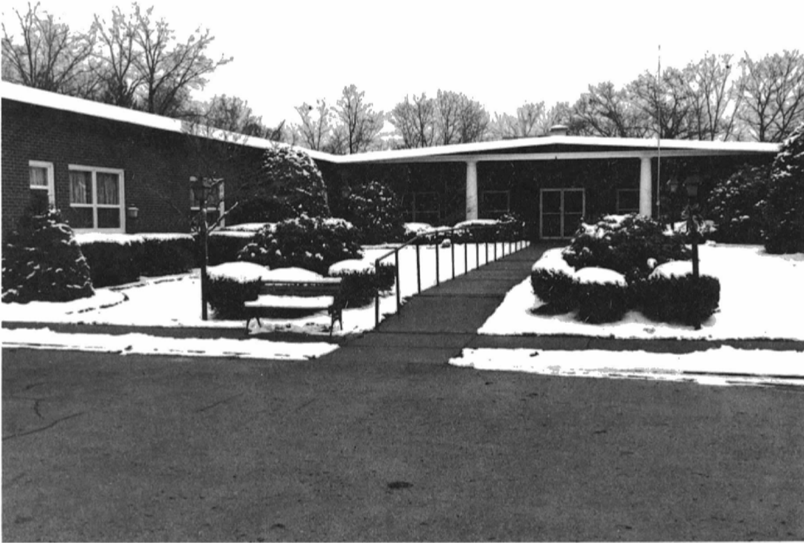
Figure 2.6 Front of Scenery Hill Manor Nursing Home
