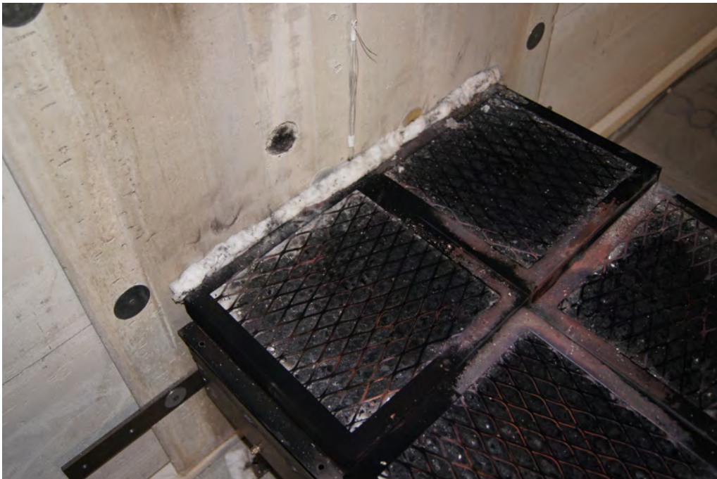
Fig. 3. Photograph of the strip of mineral wool sealing the gap.
