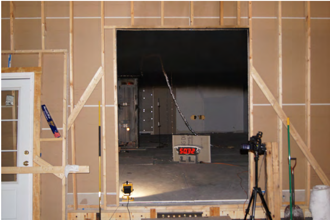
Fig. 24. Photograph of medium cabinet with 200 kW fire (Test 7).
