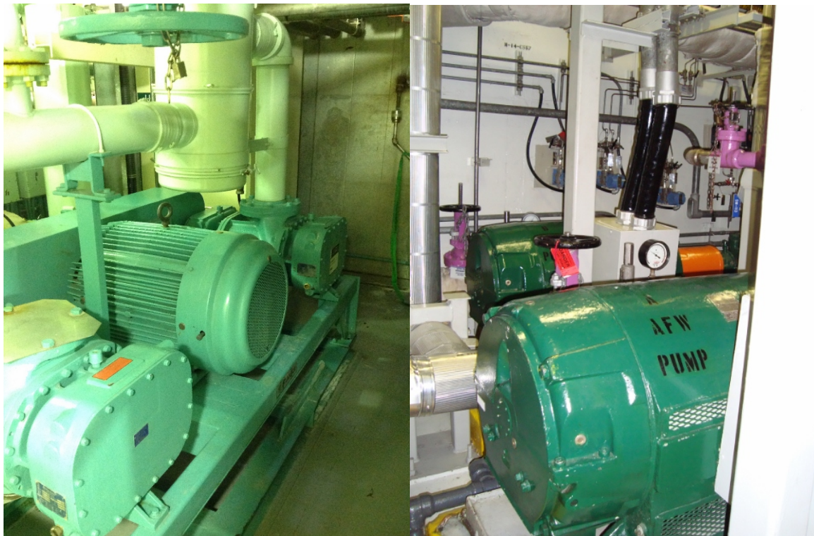
Figure 5-6 Examples of Group C motors (200 hp, 350 hp)
