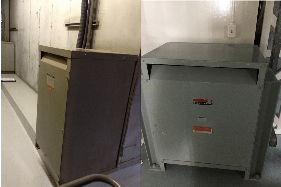
Figure 5-14 Examples of typical dry transformers, low end of range (50 kVA, 75 kVA)
