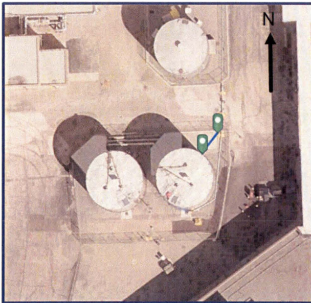
Figure 3: 2/3 Condensate Storage Tank
