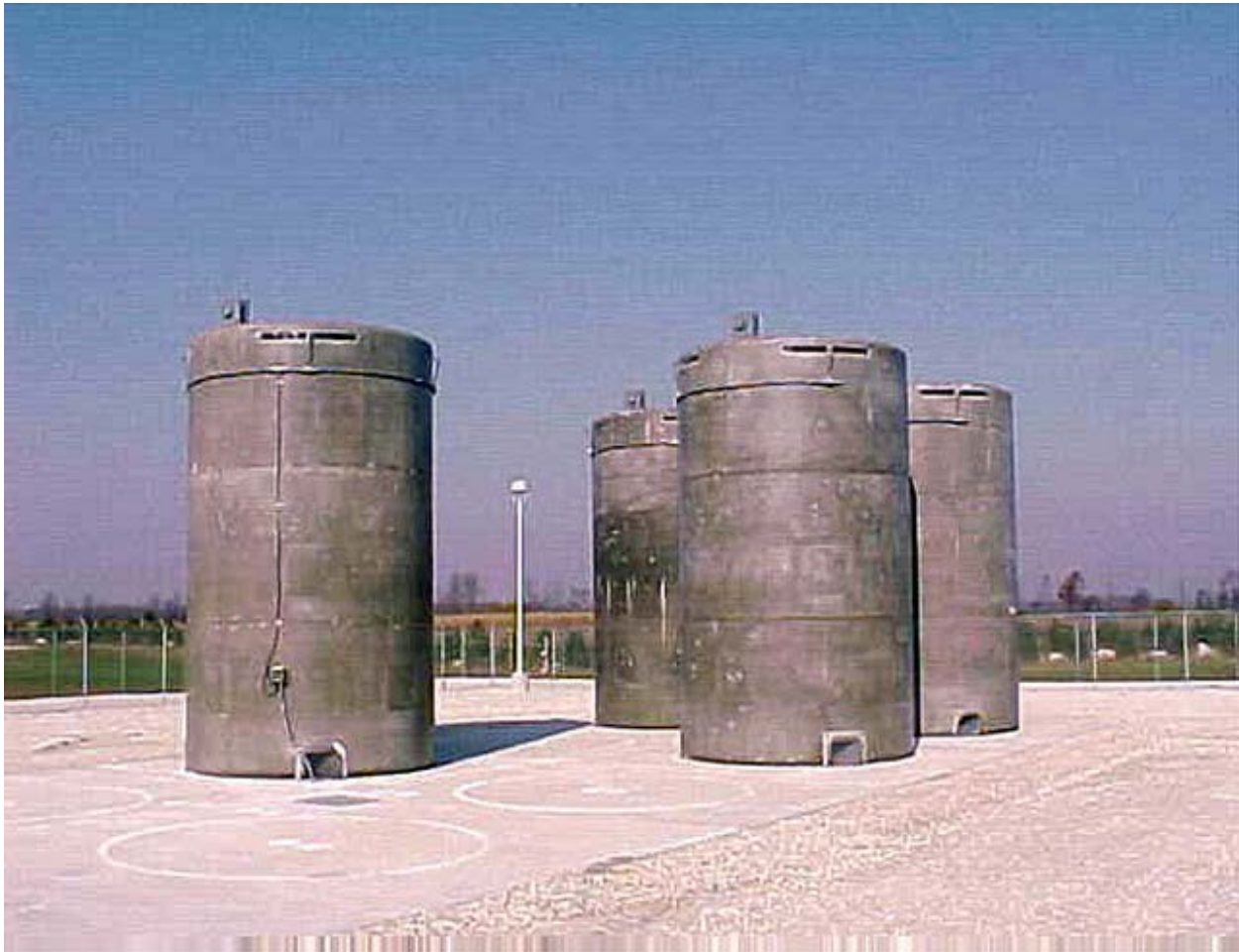
Spent Fuel Dry Cask Storage
