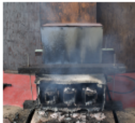
Zion Bus Duct (testing) 2016
