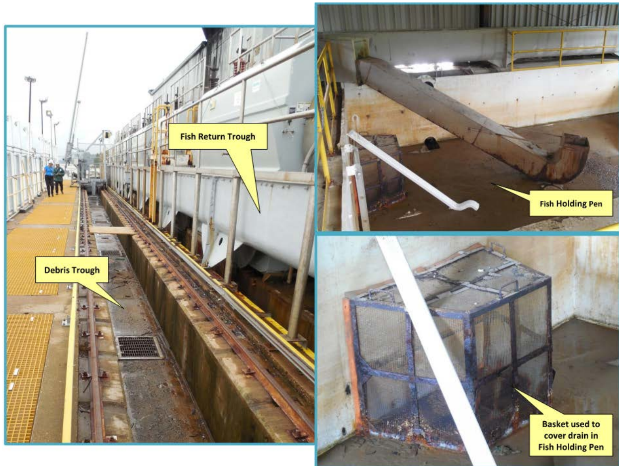
Figure 6-2. Pictures of Surry Power Station Fish Return Trough, Fish Holding Pen and Basket to Cover the Drain of Fish Holding Pen
