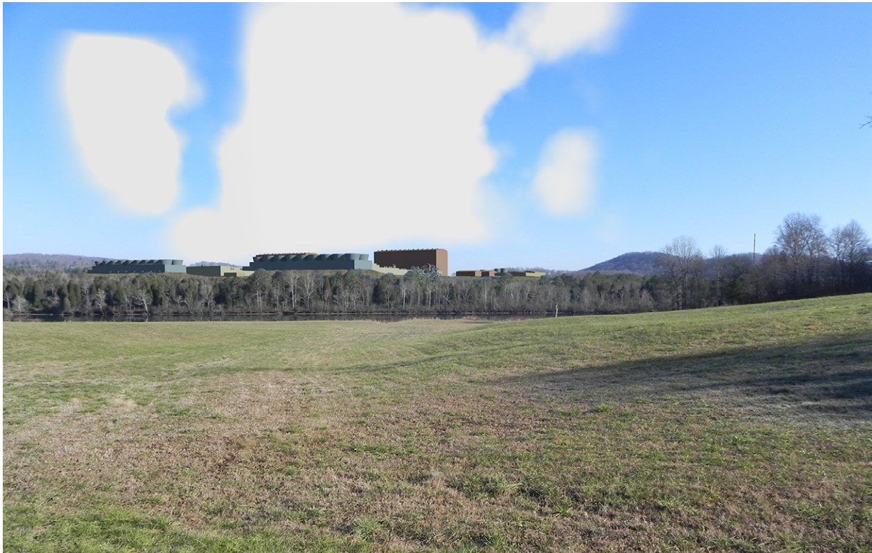
Figure 5-3 Visual Simulation of the Operating Facilities at the CRN Site Showing the Annual Average Cooling-Tower Plume. View looking south to north. (Source: TVA 2019-TN5854)
