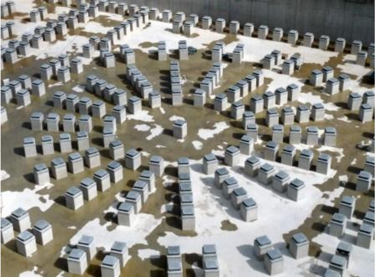
Figure 2-19 Isolators installed on the site of ITER ( http://www.iter.org )
