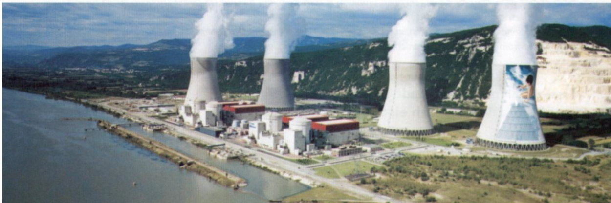
Figure 2-3 Four units of seismically isolated NPP at Cruas, France (Forni and Poggianti, 2011)
