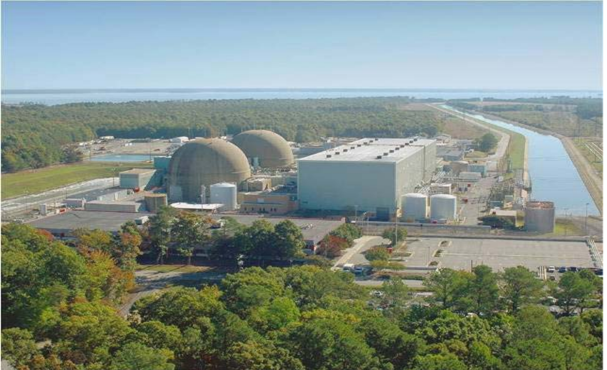
Figure E3.8-12 Post-Construction Photograph of SPS Showing Structures, Buildings, and Parking Lots Surrounded by Forest
