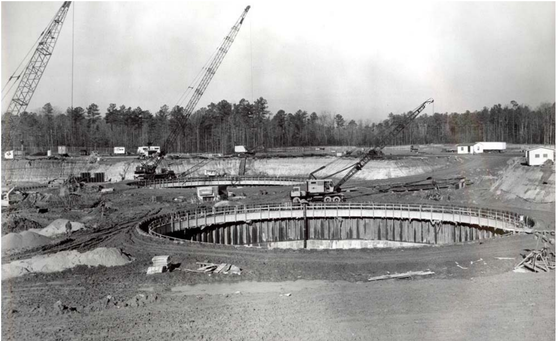
Figure E3.8-11 Construction Photograph of SPS, Showing Areas Excavated for Structures
