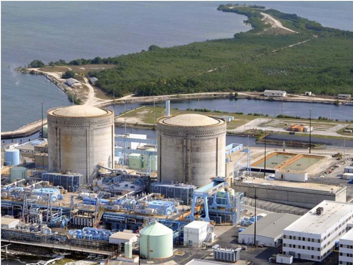
Turkey Point Nuclear Plant Units 3 and 4
