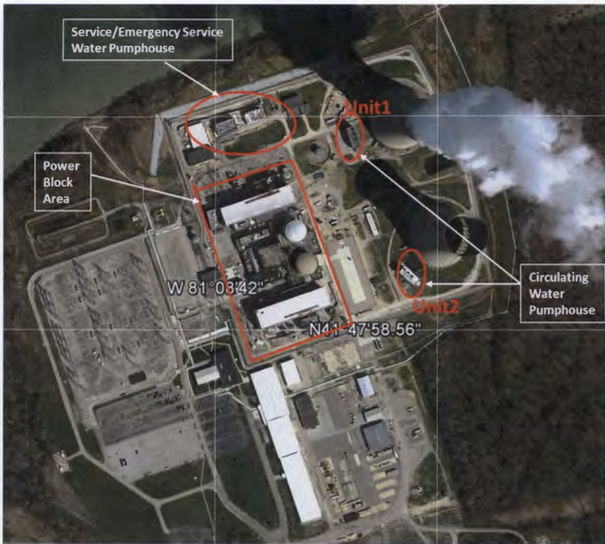
Figure 3.2-1. Perry site layout showing the Power Block and other areas (Service/Emergency Service Pump House and Circulating Water Pump House for Unit 1 and Unit 2), where the 83 door locations were evaluated in LIP analysis.
