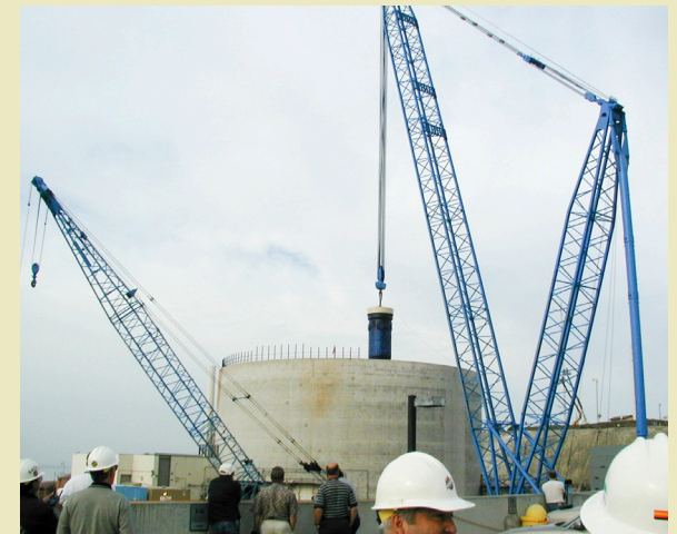
Images of decommission job at San Onofre Unit 1 in California.
