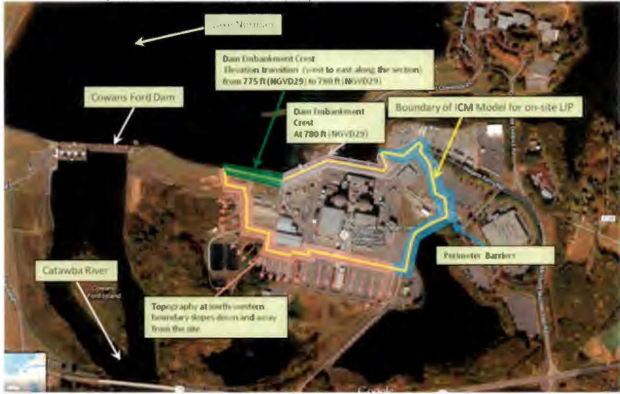
Figure 3.2.2-1 Site layout for the McGuire Nuclear Station, Units 1 and 2 (from FHRR staff assessment).
