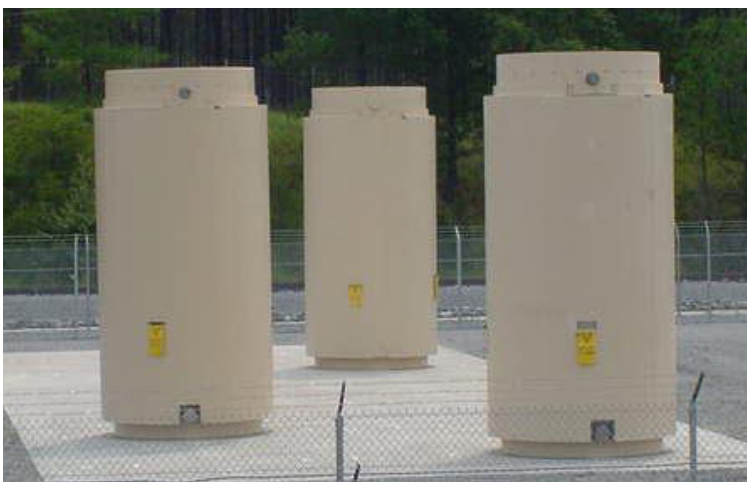
Portable spent fuel storage casks sit on a storage pad. (Courtesy: Holtec International)
