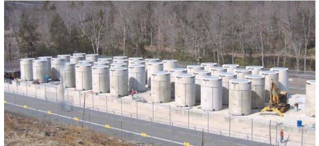
Loaded spent fuel storage casks are in place on storage pad at the Haddam Neck Plant in Meriden, CT. (Courtesy: Connecticut Yankee)
