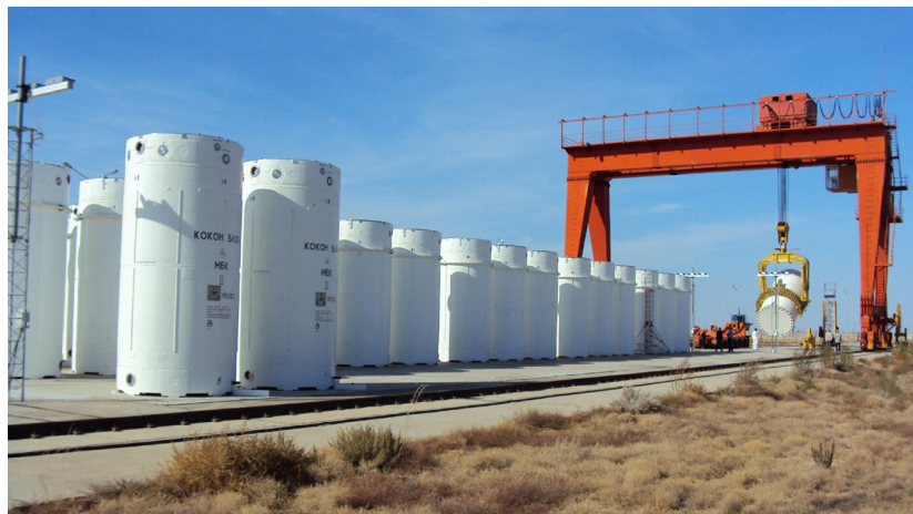
At right, a dry storage cask recently loaded with spent fuel is lifted from a horizontal transporter to be placed on a specially designed storage pad. (Courtesy: Sandia National Laboratories)
