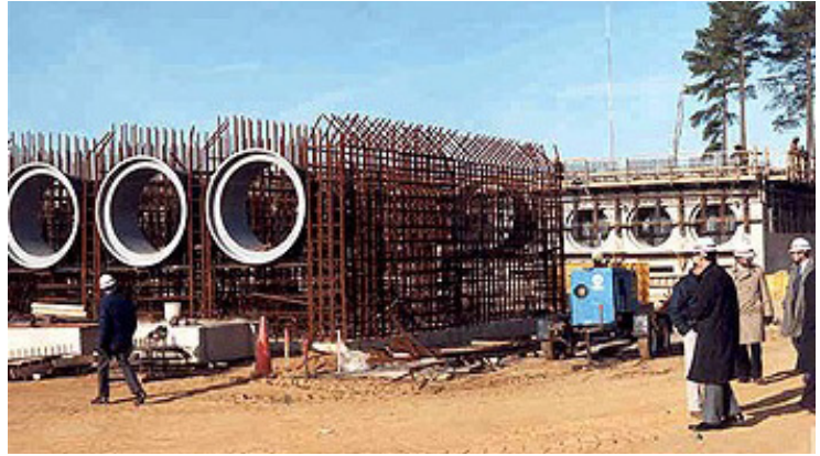
NUHOMS horizontal spent fuel storage system under construction at the Calvert Cliffs Nuclear Power Plant in Lusby, MD.
