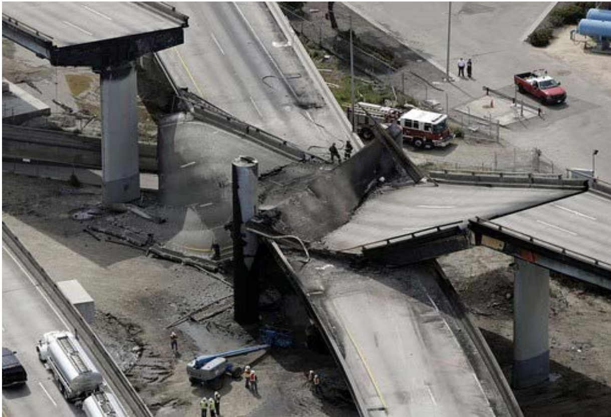
Figure 5.14. Roadway Configuration after the MacArthur Maze Fire (photo from MAIT Report, CHP 2007a)
