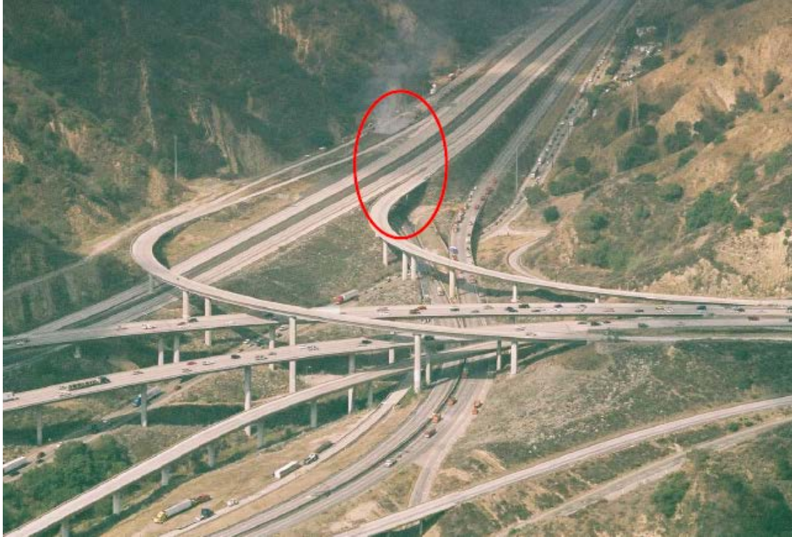
Figure 5.16. Aerial View of Roadway Configuration Showing Location of Newhall Pass Tunnel (image extracted from the CHP MAIT report [CHP 2007b])
