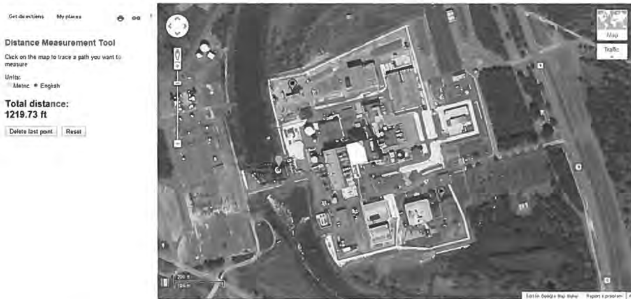
Figure 3: FLEX Storage Pad location for tornado wind protection
