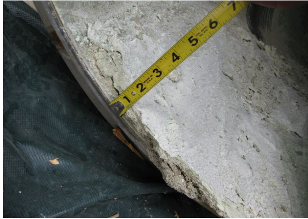
May 27, 2016 Inlet Transition Elbow
