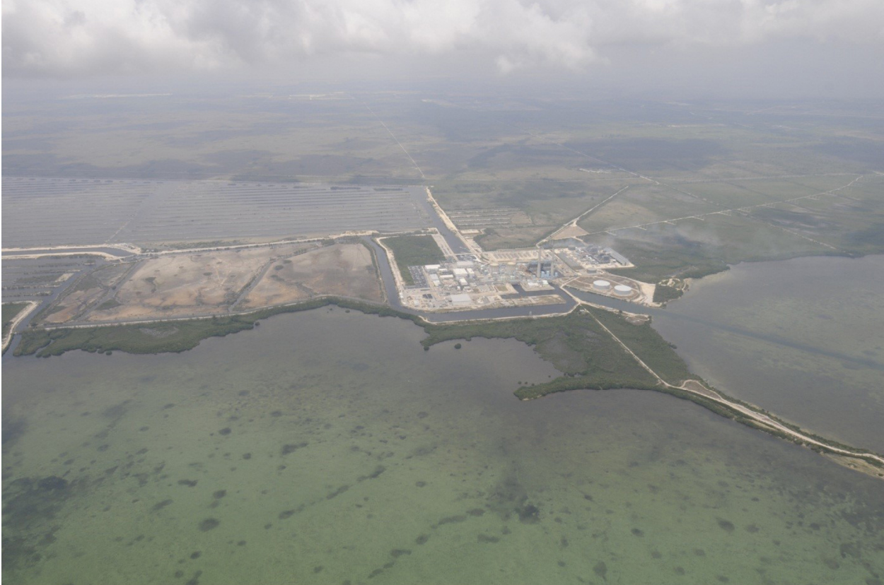
Figure 2-3. Oblique Aerial Photograph of the Proposed Units 6 and 7 Plant Area and Surrounding Area (Adapted from FPL 2014-TN4058)
