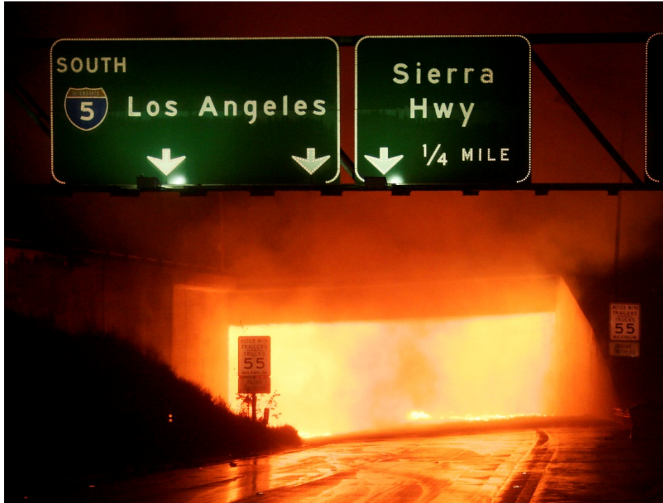
Figure S.1. Newhall Pass Tunnel Entrance at 10/13/2007 2:47 a.m. (photo from MAIT Report, CHP 2007, reprinted with permission.)
