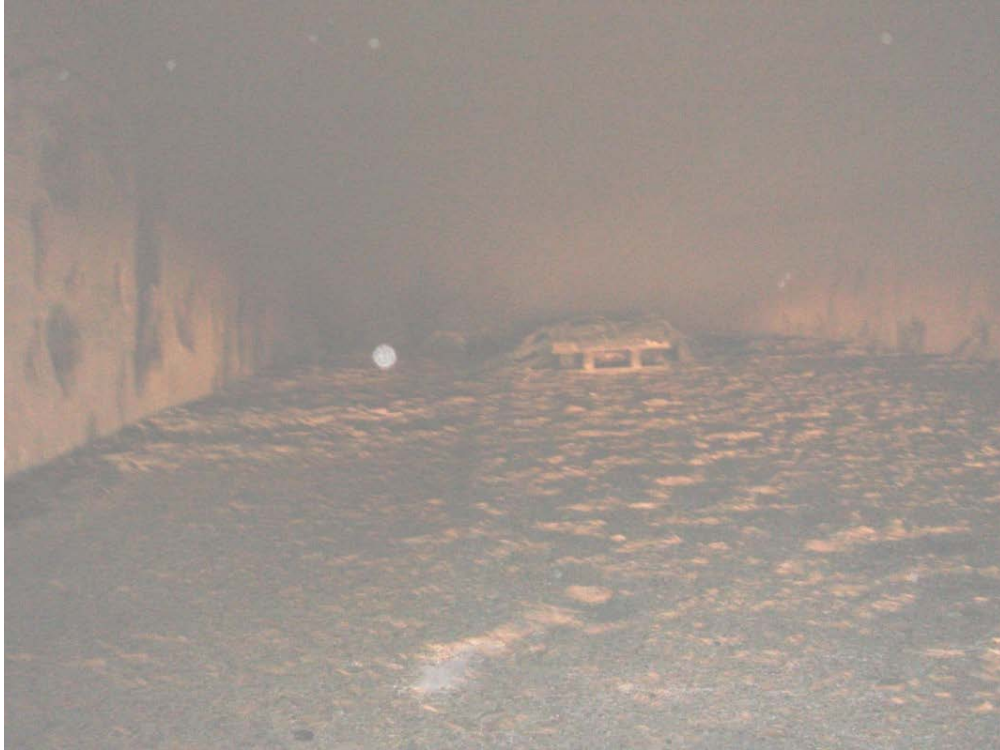
Figure 2.5. Newhall Pass Tunnel Entrance at 10/13/2007 4:04 a.m. (photo from MAIT Report, CHP 2007, reprinted with permission.) 1
