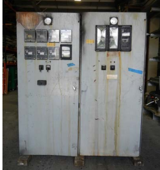
Figure 4.10-3. SWGR Test 3 Exterior Damage
