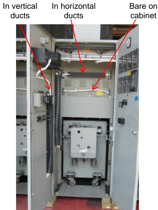
Figure 4.4-1. SWGR Cabinet Combustible Load
