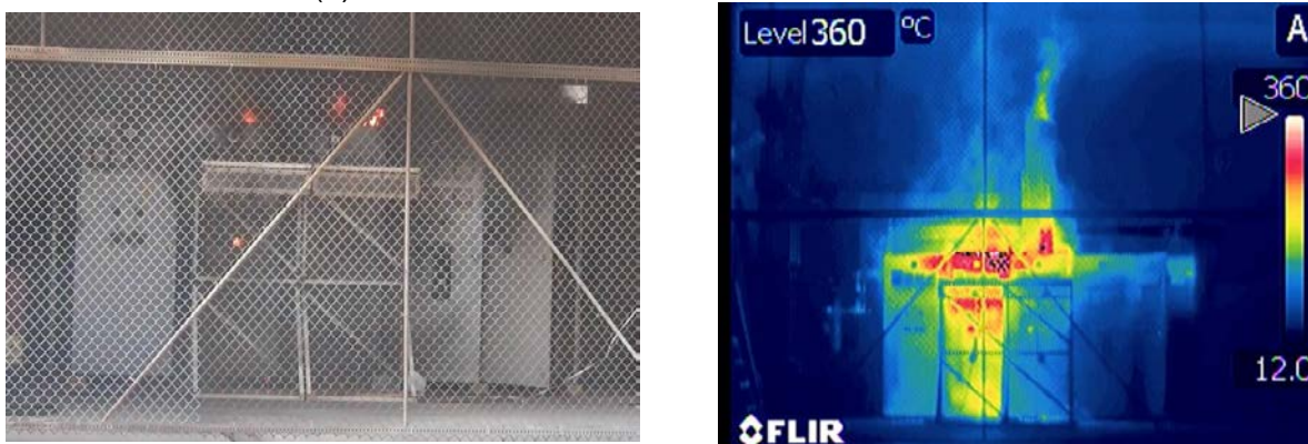
Figure 5.5-2. SWGR Test 4 Thermal Image Ensuing Fire
