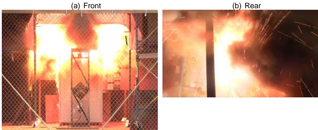
Figure 2.11-2. DP Test 4 Arc Flames
