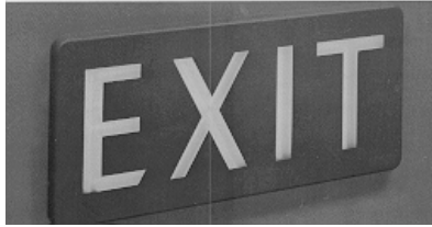
Figure G–3. Self-Luminous Exit Sign. Certain self-luminous, tritium exit signs can be possessed under 10 CFR 31.5. (Typical devices initially contain 25 curies of tritium per sign.)
