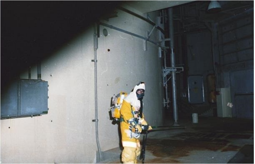
Above: First entry into the reactor building (shown) occurred on July 23, 1980. Heavy duty outerwear provided high-energy beta ray protection. Below: Water level in the basement of the reactor building reached the first stairwell landing indicating about 8 feet of water accumulation. One-third of this highly radioactive water came from leakage of non-radioactive river water coolant from a leaking reactor building air-handling cooler.
