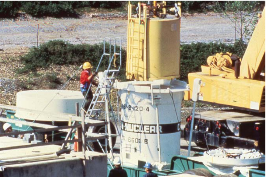
Spent EPICOR II resin liner inside the shielded transfer cask (yellow) being lowered into a shipping cask.
