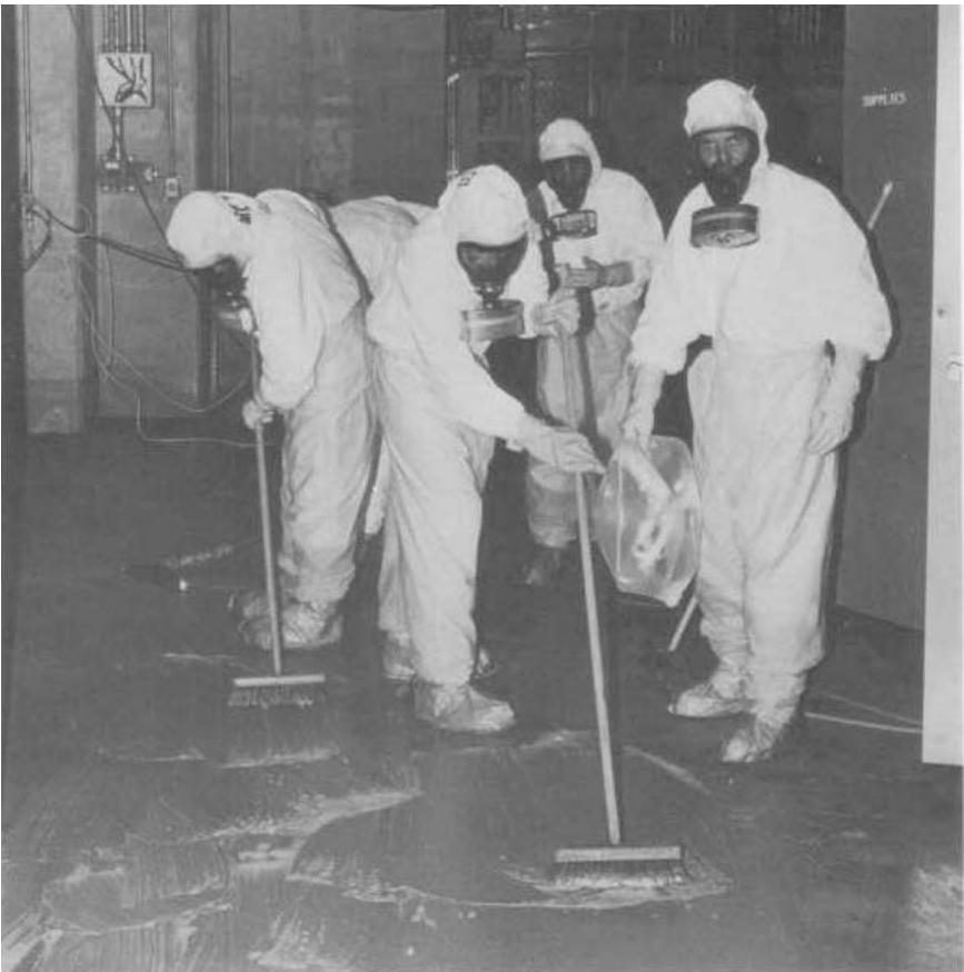
Workers decontaminating the auxiliary building using the manually applied scrubbing method.
