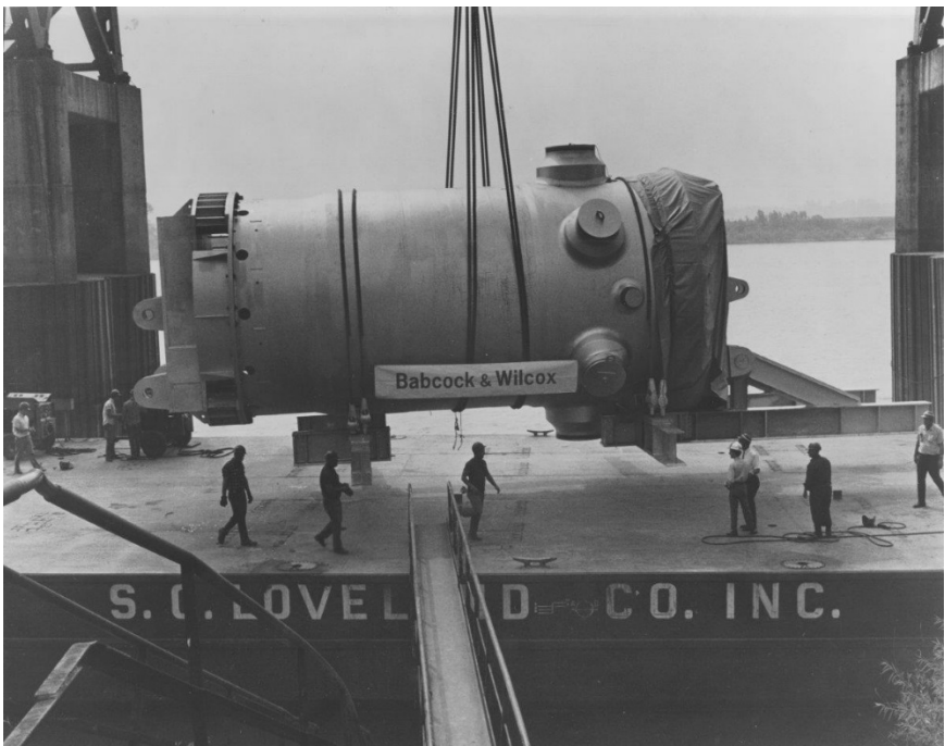
The reactor pressure vessel on its way for installation at TMI-2. (This photo was taken either during the loading operation at the Babcock and Wilcox fabrication facility in Mount Vernon, Indiana, or during the unloading near Havre de Grace, Maryland.)
