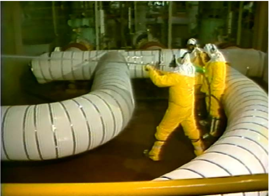
Decontamination using high-pressure spray.
