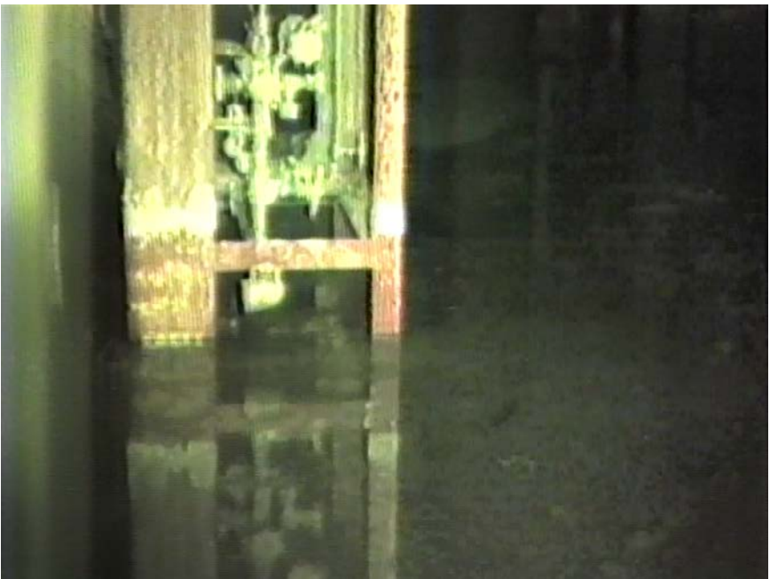
The basement in the reactor building contained about 8 feet of highly contaminated water. The submerged demineralizer system started processing basement water on September 9, 1981.
