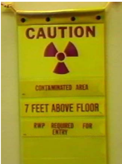
A radiation work permit (RWP) was required to access contaminated ceiling areas above the clean areas of the auxiliary building main corridors.
