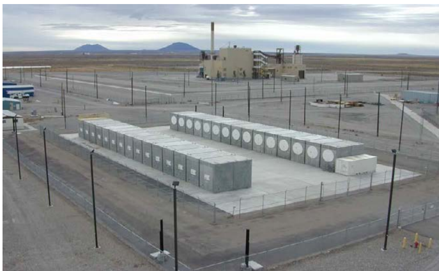
TMI-2 independent spent fuel storage installation located at INEL for interim storage of the TMI-2 core debris.
