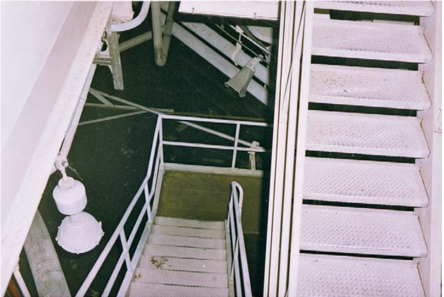
Above: First entry into the reactor building (shown) occurred on July 23, 1980. Heavy duty outerwear provided high-energy beta ray protection. Below: Water level in the basement of the reactor building reached the first stairwell landing indicating about 8 feet of water accumulation. One-third of this highly radioactive water came from leakage of non-radioactive river water coolant from a leaking reactor building air-handling cooler.
