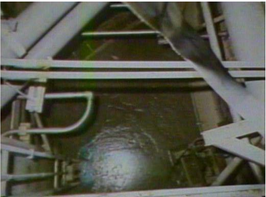
Highly radioactive sludge on the basement floor of the reactor building as viewed from an upper level. A robotic desludging system was used to vacuum the 40 percent of the basement floor area that was accessible to the robot.
