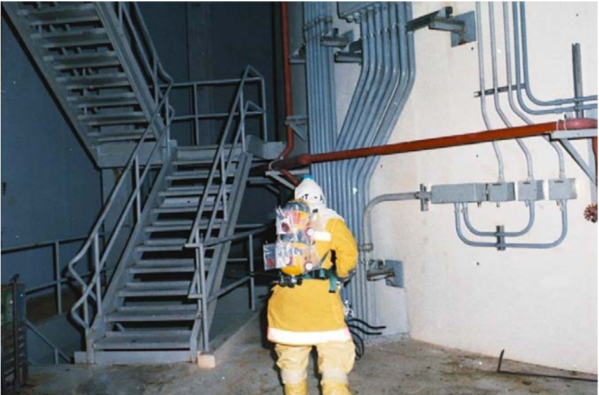
First entry into the reactor building (shown) occurred on July 23, 1980. Heavy duty outerwear provided beta ray protection.
