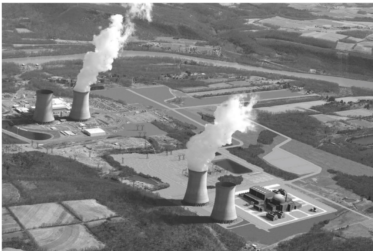
Figure 3-2. The BBNPP Site with Existing SSES Units 1 and 2 at Left and Proposed BBNPP Unit Superimposed at Right (PPL Bell Bend 2013-TN3377)
