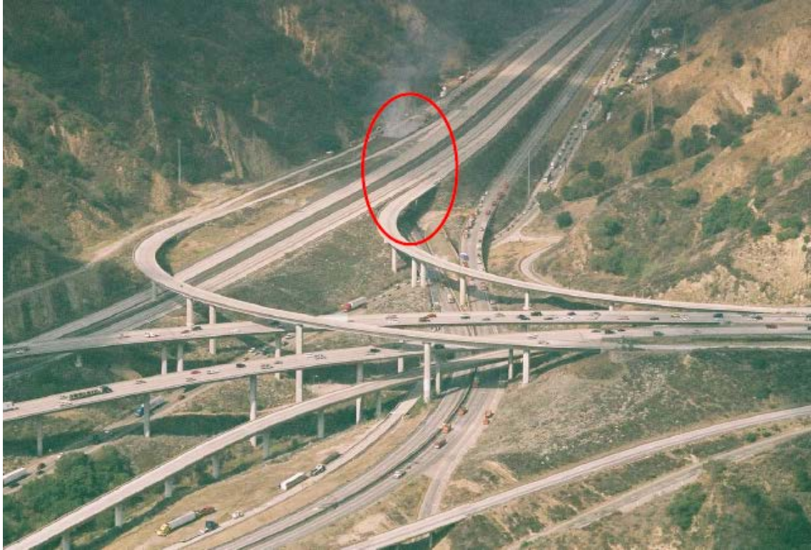
1 2 Figure 5.16. Aerial View of Roadway Configuration Showing Location of Newhall Pass Tunnel 3 (image extracted from the CHP MAIT report [CHP 2007b]) 4
