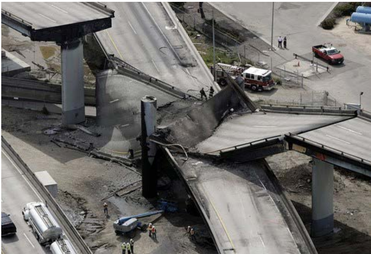
15 16 Figure 5.14. Roadway Configuration after the MacArthur Maze Fire (photo from MAIT Report, 17 CHP 2007a) 18
