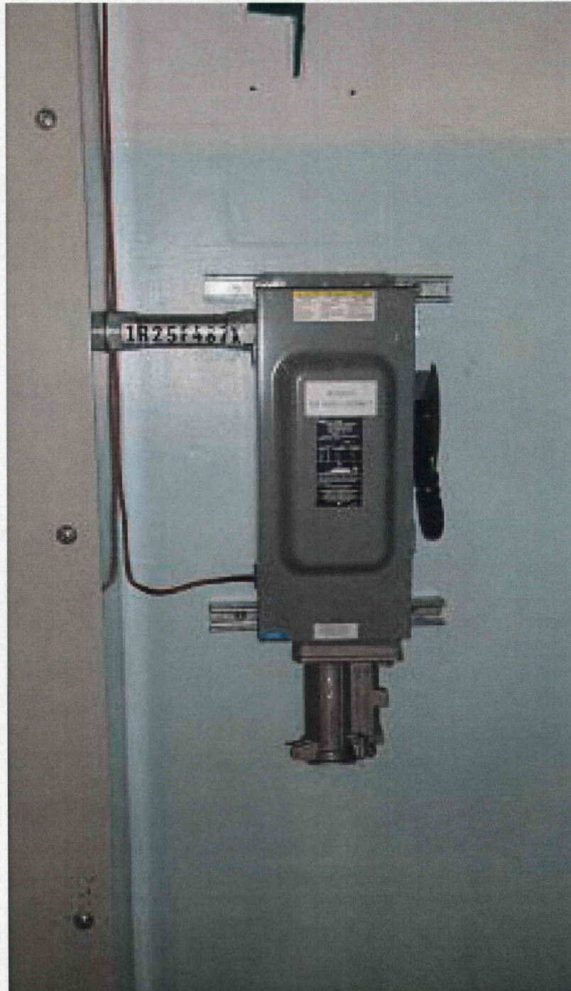
FLEX Alternate CRD Injection Pump Disconnect
