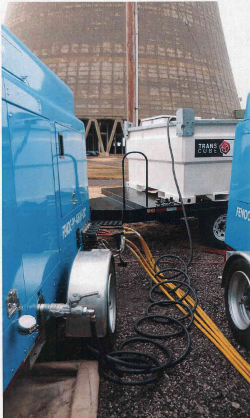
Fuel oil line connections from Transcube to 4160 Vac Generator during FLEX Lake Water Pump Testing
