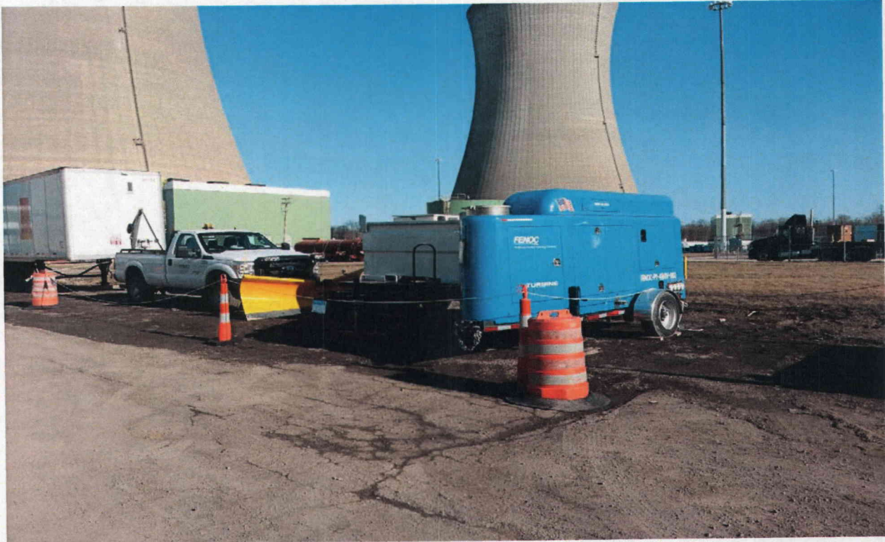
Debris removal truck, Transcube and Flex generator staged south of ESW Pumphouse between pump tests
