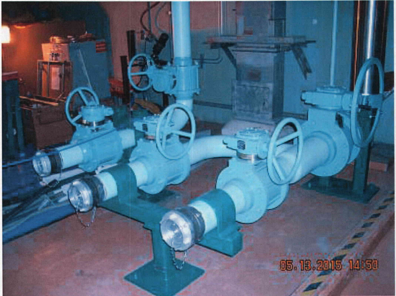
ESW A (foreground) and FPCC (rear) Tie Ins
