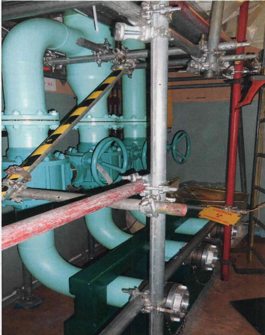
FPCC Tie In
