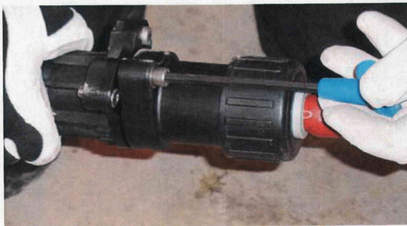
Detail of cable connection being made
