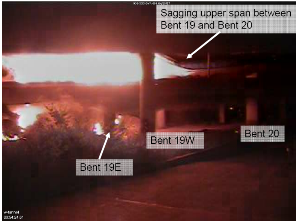
1 2 Figure S.1. MacArthur Maze Fire at +16.7 Minutes (WTP Video Image at 03:54:24.61 PDT, 3 photo from MAIT Report, CHP 2007, reprinted with permission.) 4
