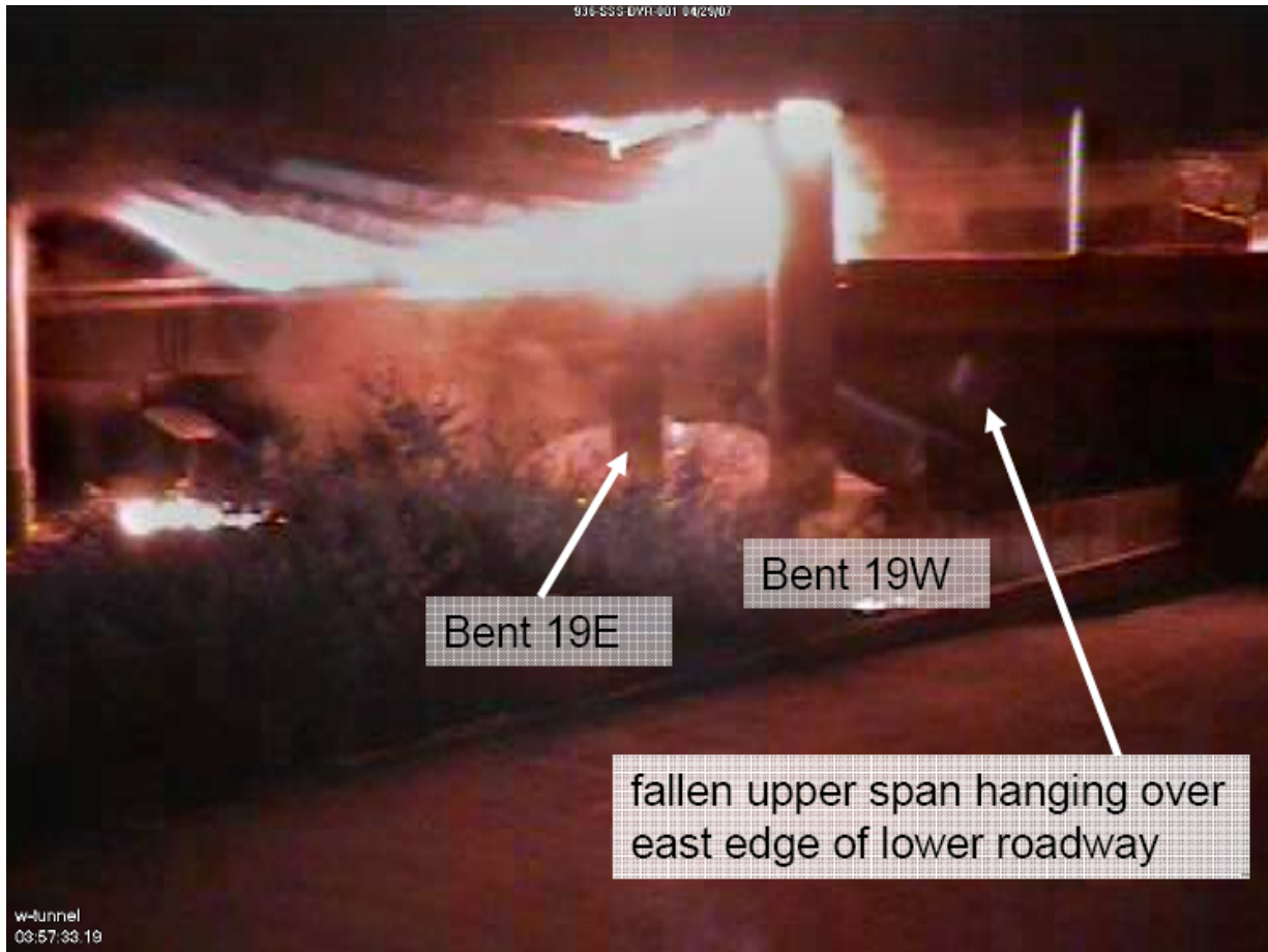
1 2 Figure 2.4. MacArthur Maze Fire at +19.8 Minutes (WTP video image at 03:57:33.19 PDT, 3 photo from MAIT Report, CHP 2007, reprinted with permission.) 4 5 The slow gradual descent of the Bent 19 end of the second I-580 span to the lower roadway is 6 clearly shown in the WTP video. The partial collapse of this span appears to be complete by 7 37.3 minutes into the fire, as illustrated in Figure 2.5. This image shows that the fire has self- 8 extinguished in the region between Bent 18 and the point where the upper span contacts the 9 roadway. The fire is confined to a relatively narrow region near Bent 19, between the ends of 10 the two fallen I-580 spans.
