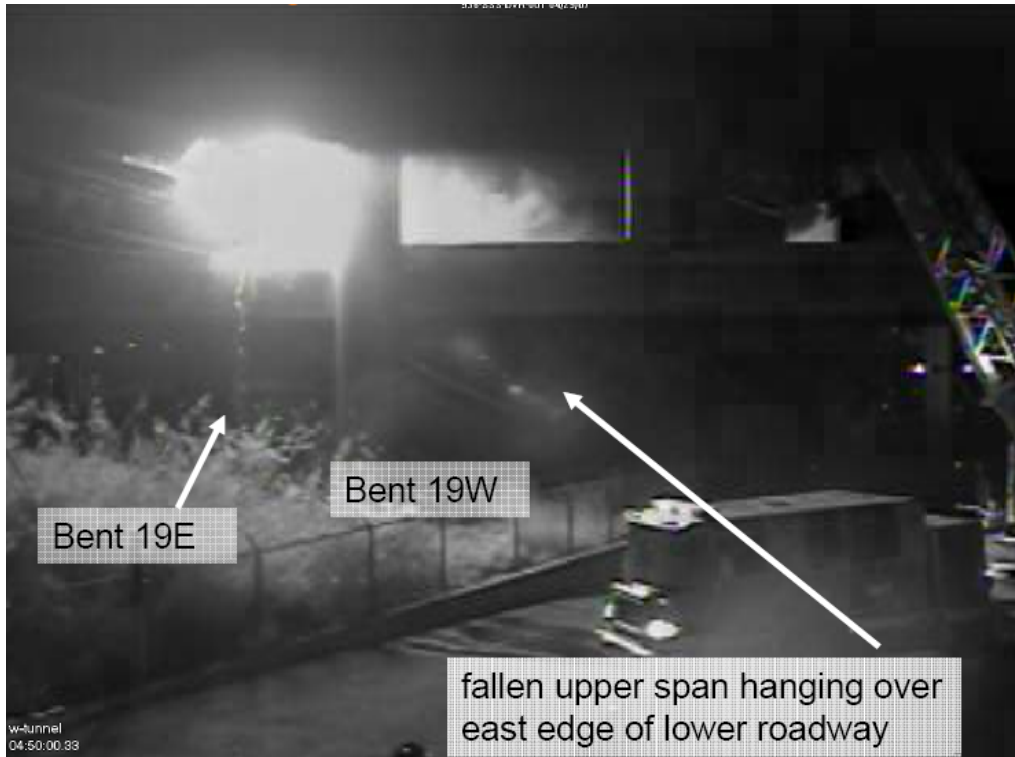
1 2 Figure 2.6. MacArthur Maze Fire at +72.3 Minutes (WTP video image at 04:50:00.33 PDT, 3 photo from MAIT Report, CHP 2007, reprinted with permission.) 4
