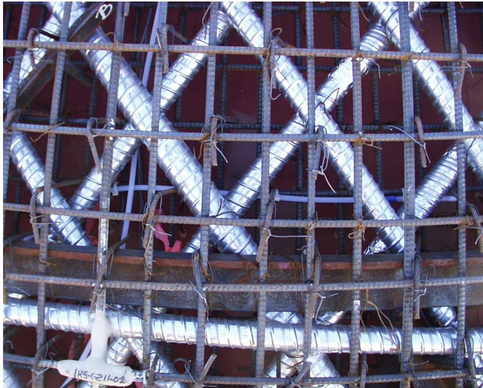
Figure 2-10 Tendon ducts in 1:4-scale PCCV (silver colored tubes) along with traditional rebar
