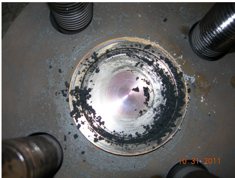
Figure 3-37. Photograph showing the disintegration of the tested EPDM O-ring when an attempt was made to remove the O-ring from the groove.
