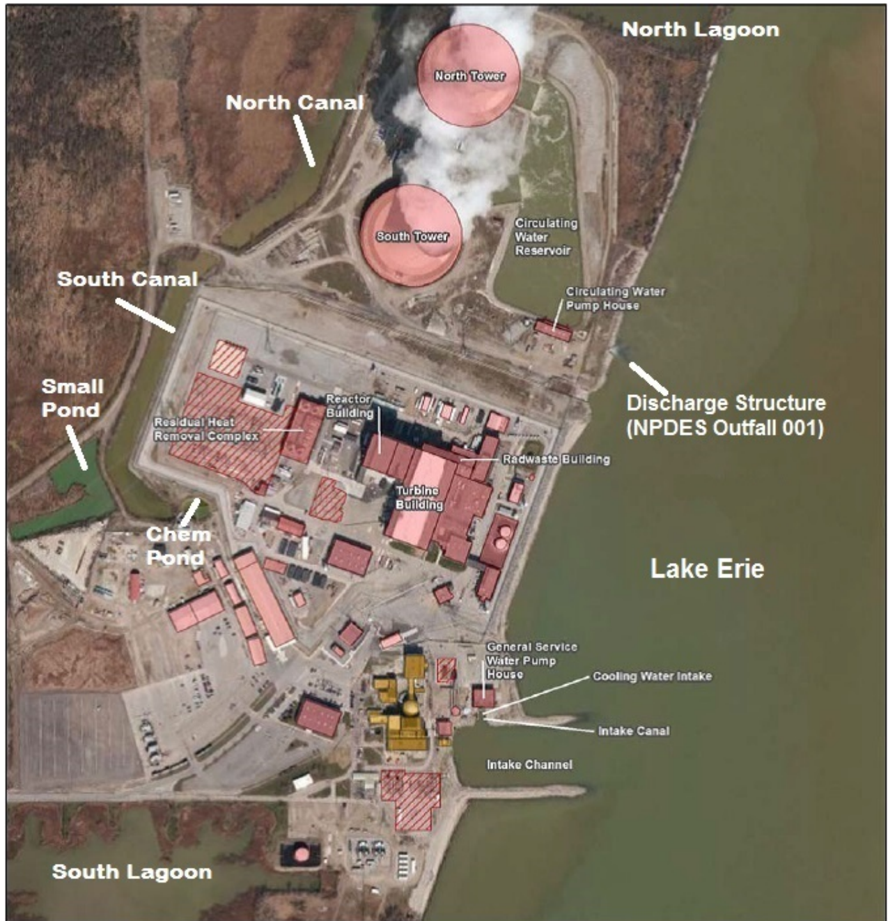
1 Figure 3–5. Fermi 2 Cooling Water Supply Facilities and Major Surface Water Features
