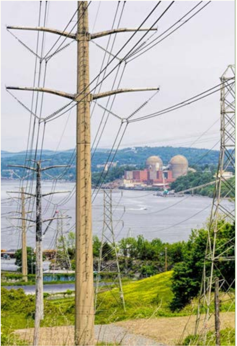
The Indian Point nuclear power plant located in Buchanan, NY.
