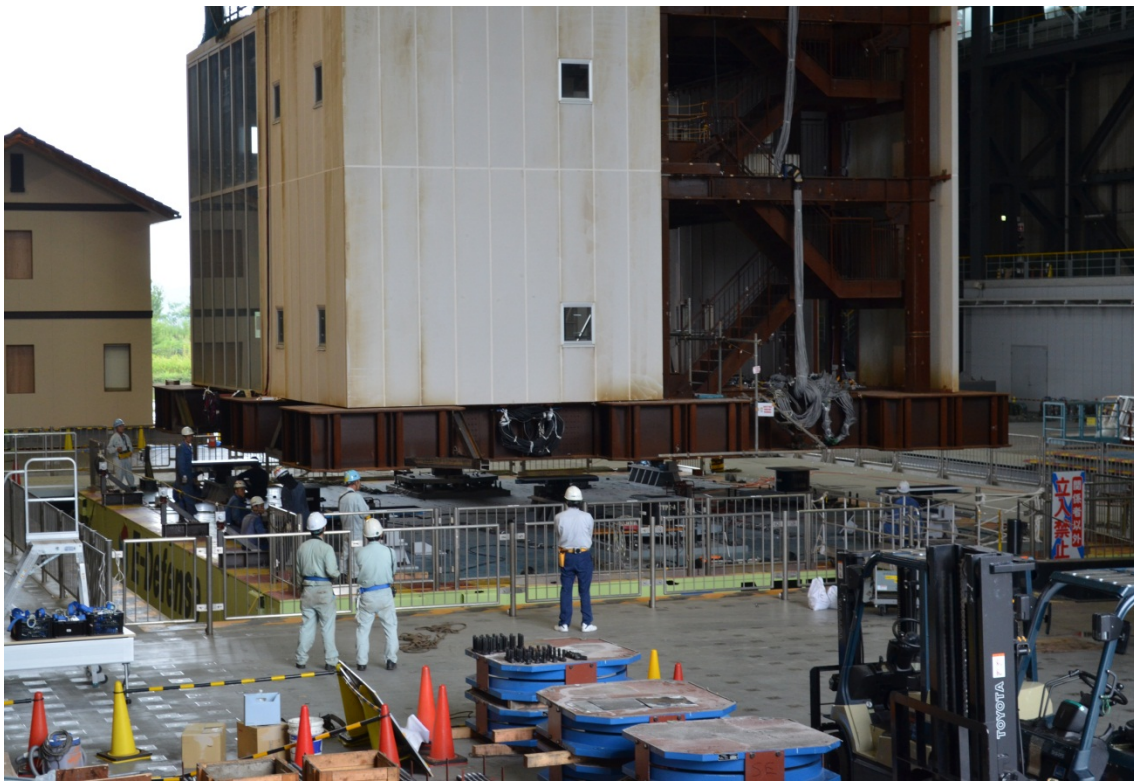
Figure 4-15 Lowering the testbed building over the isolation system
