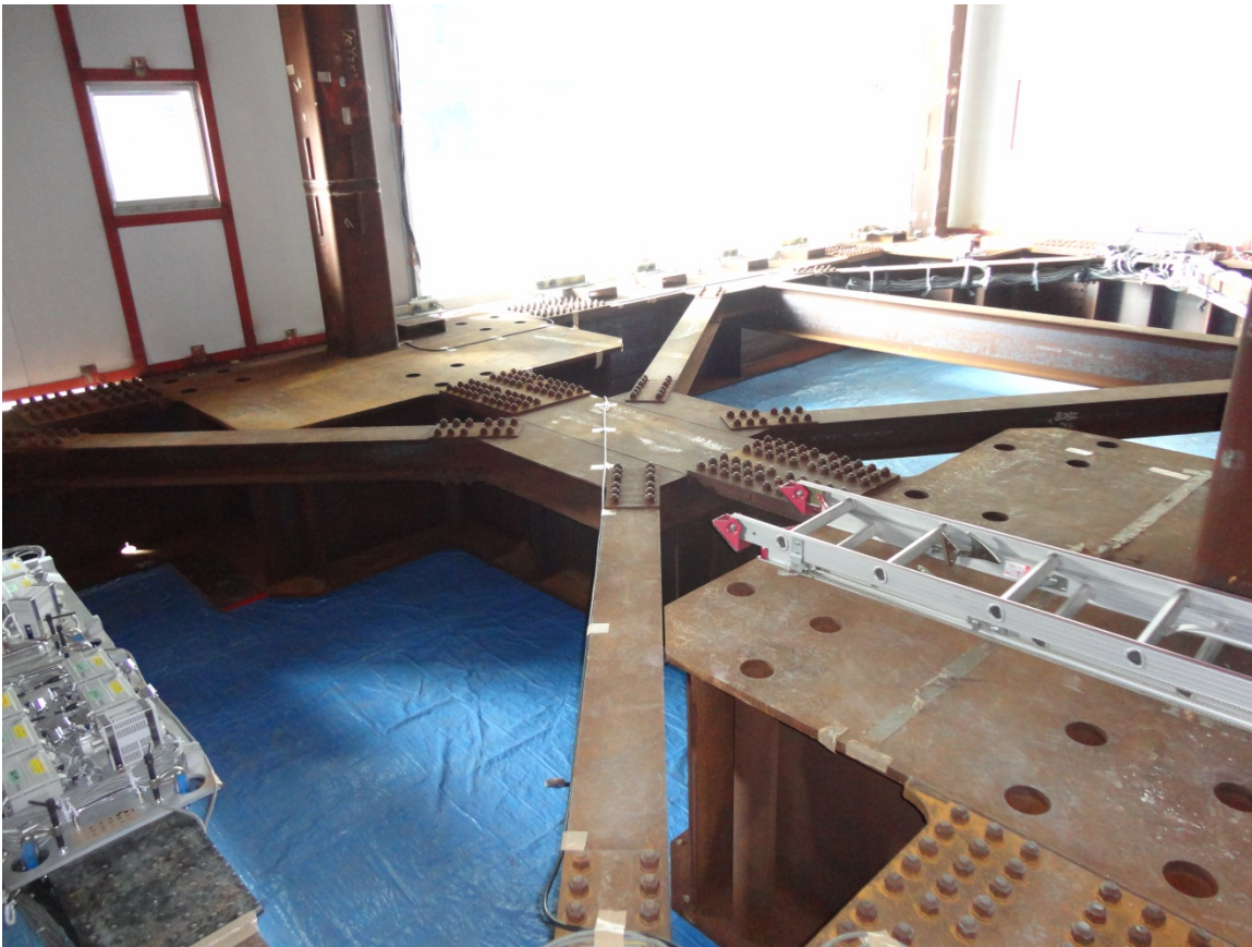
Figure 2-6 Horizontal braces at base level
