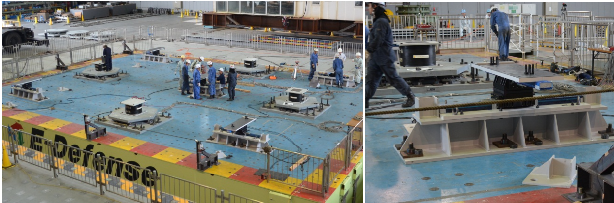
Figure 4-14 Installing the LR bearings to the connecting assemblies and the CL bearings to the simulator platform
