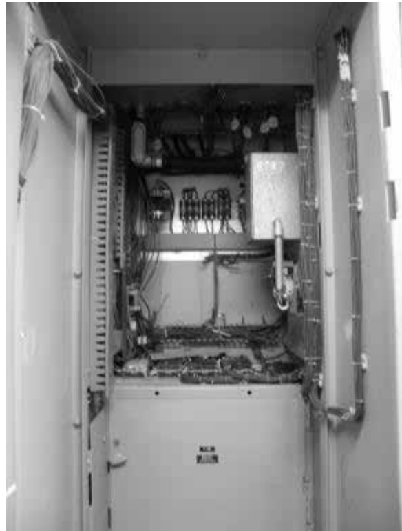
1 Figure 2-3. Photographs of the internal wiring of typical switchgear enclosures.
