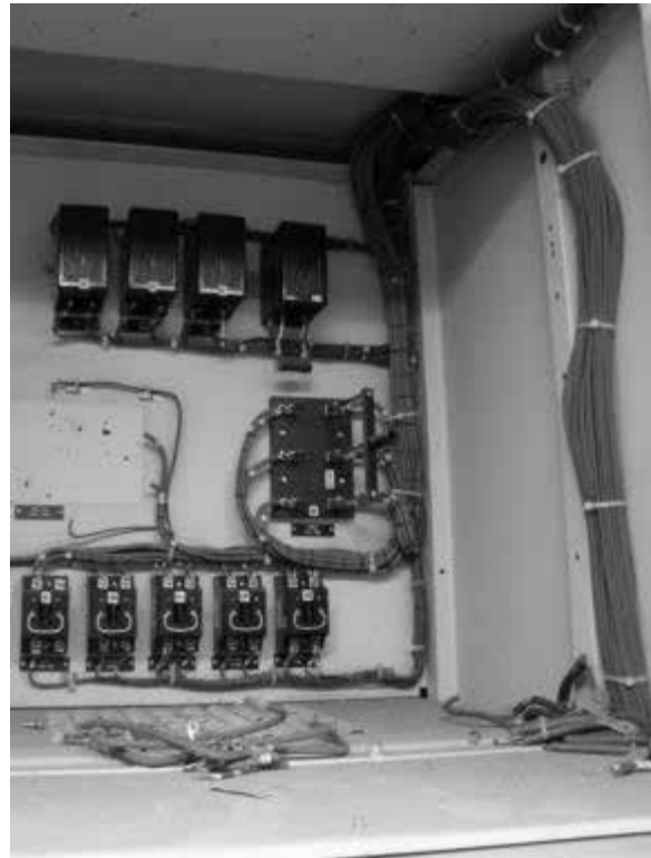
1 Figure 2-4. Photographs of the internal wiring of typical motor control centers.
