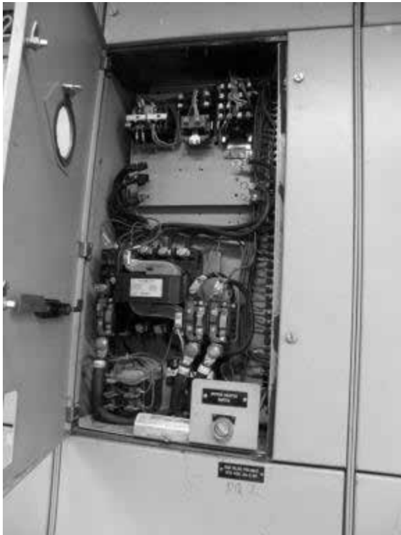
1 Figure 2-4. Photographs of the internal wiring of typical motor control centers.
