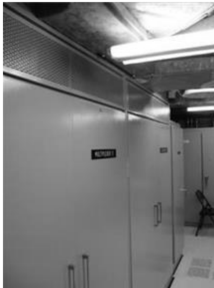
7 8 9 Figure C-17 10 Auxiliary Shutdown Panels – Large Enclosure (Closed) 11
