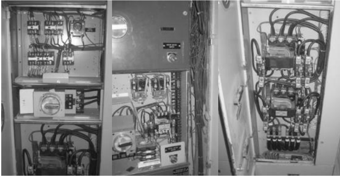
Figure C-12 Internal Views of MCC Cubicle
