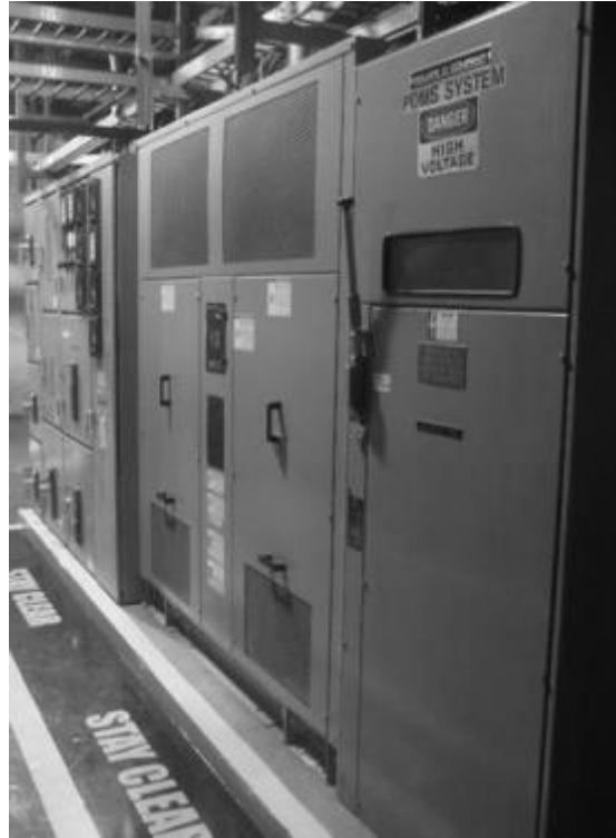
Figure C-5 Front View of Load Center (Disconnect Switch)
