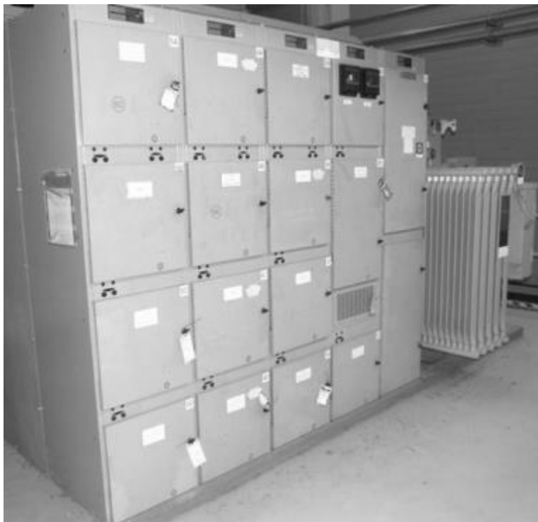
Figure C-7 Load Center (Left) with Oil-Cooled Transformer (Right)
