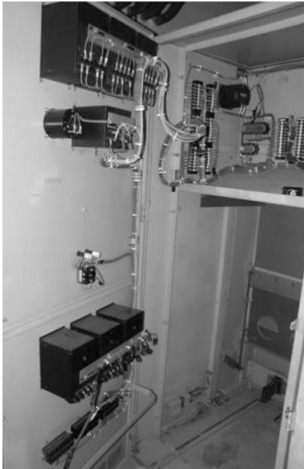
Figure C-3 Internal Views of Medium Voltage Switchgear
