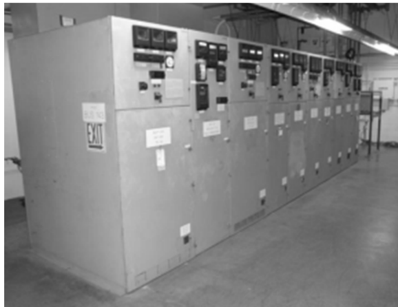
Switchgear Bank
