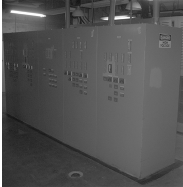
7 8 9 Figure C-17 10 Auxiliary Shutdown Panels – Large Enclosure (Closed) 11
