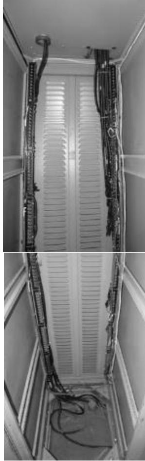
4 Figure 4-2 5 Cropped Photo of Electrical Enclosure with Bundled Panel Wiring and Cable, Limited 6 Combustible Loading, and No Ignition Sources
