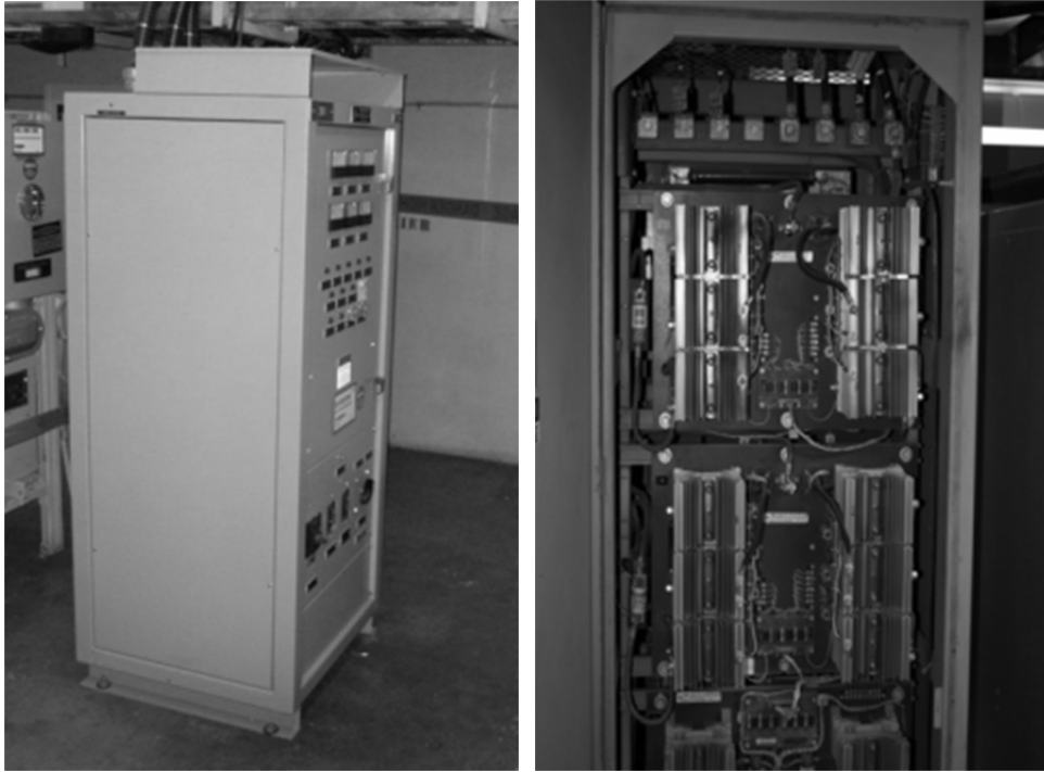
10 Figure 3-5 11 A Typical Inverter Cabinet (Exterior – Left, Interior – Right)
